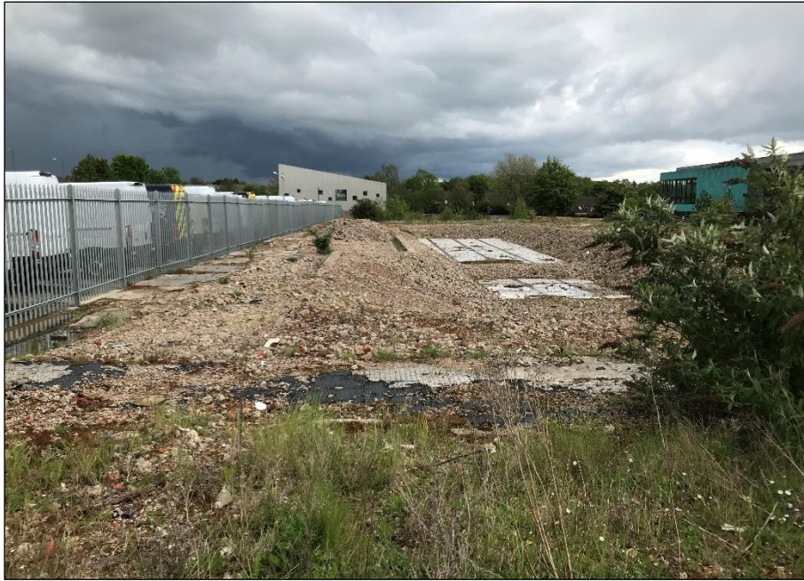
Plate 6. Tiled area and surrounding loose hardcore (looking east)
