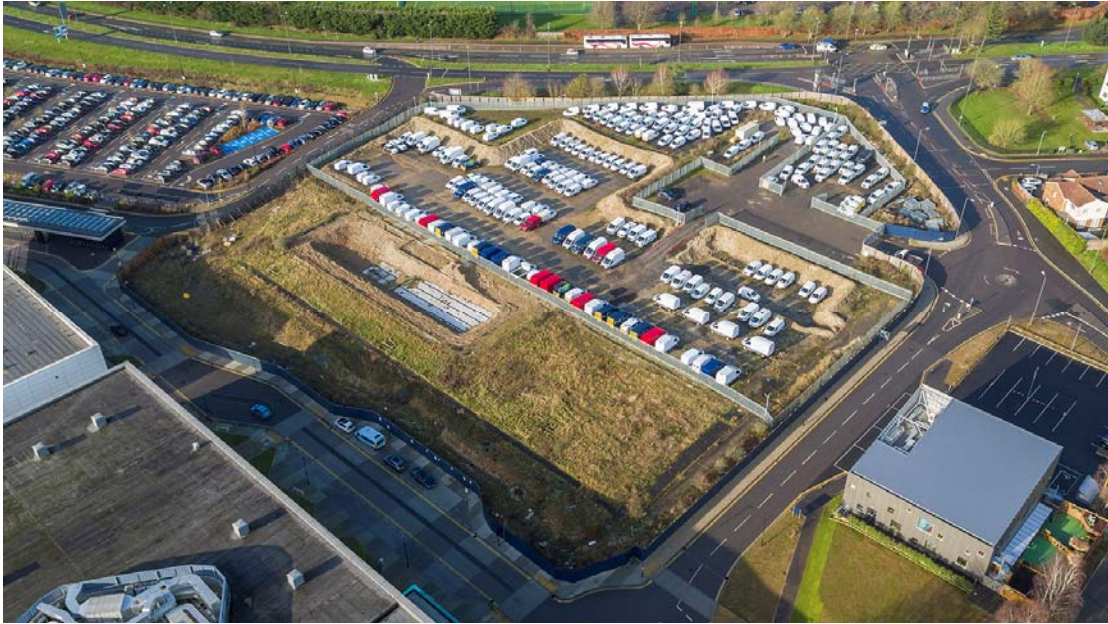
Aerial view looking North West
