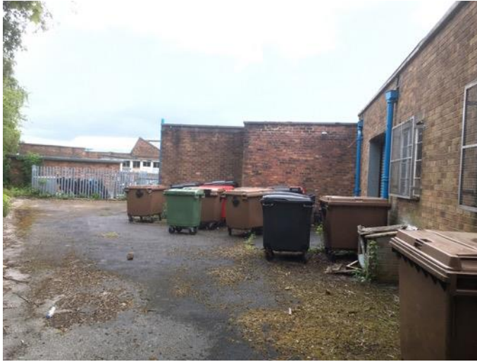
Photo of rear of existing building
