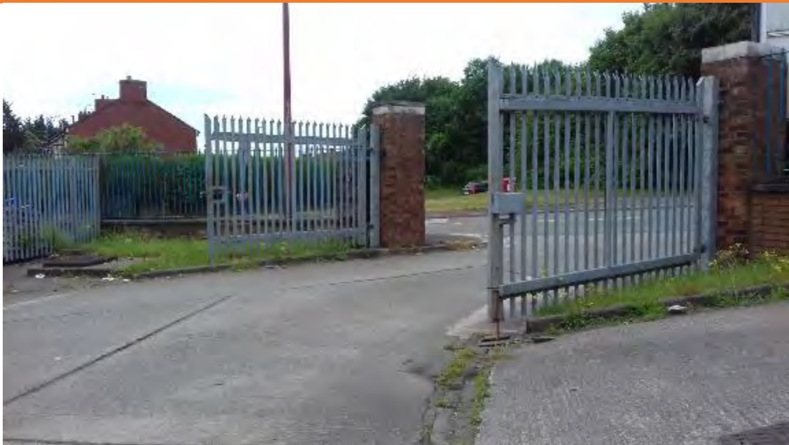
PLATE 6: SITE ENTRANCE IN WEST OF SITE
