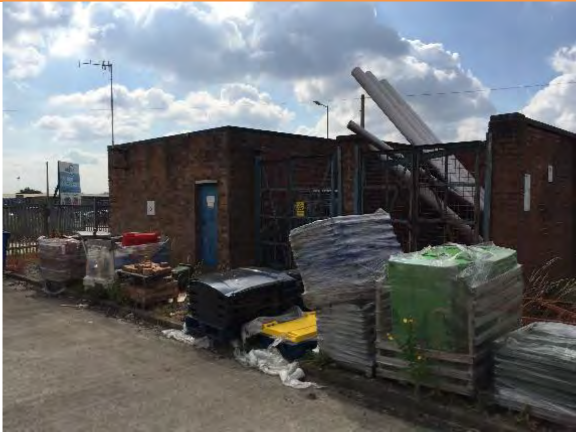
PLATE 3: ELECTRICITY SUBSTAION IN SOUTH-EAST OF SITE
