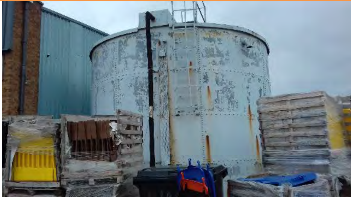
PLATE 13: WATER STORAGE TANK
