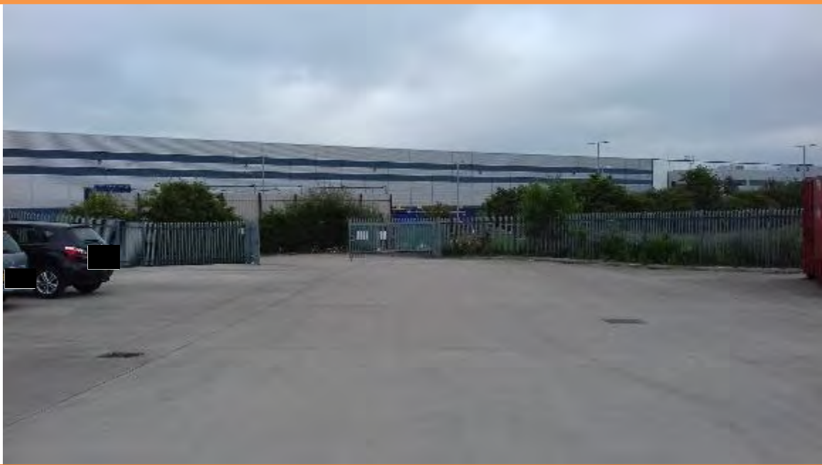
PLATE 11: VIEW OF NORTH OF THE SITE
