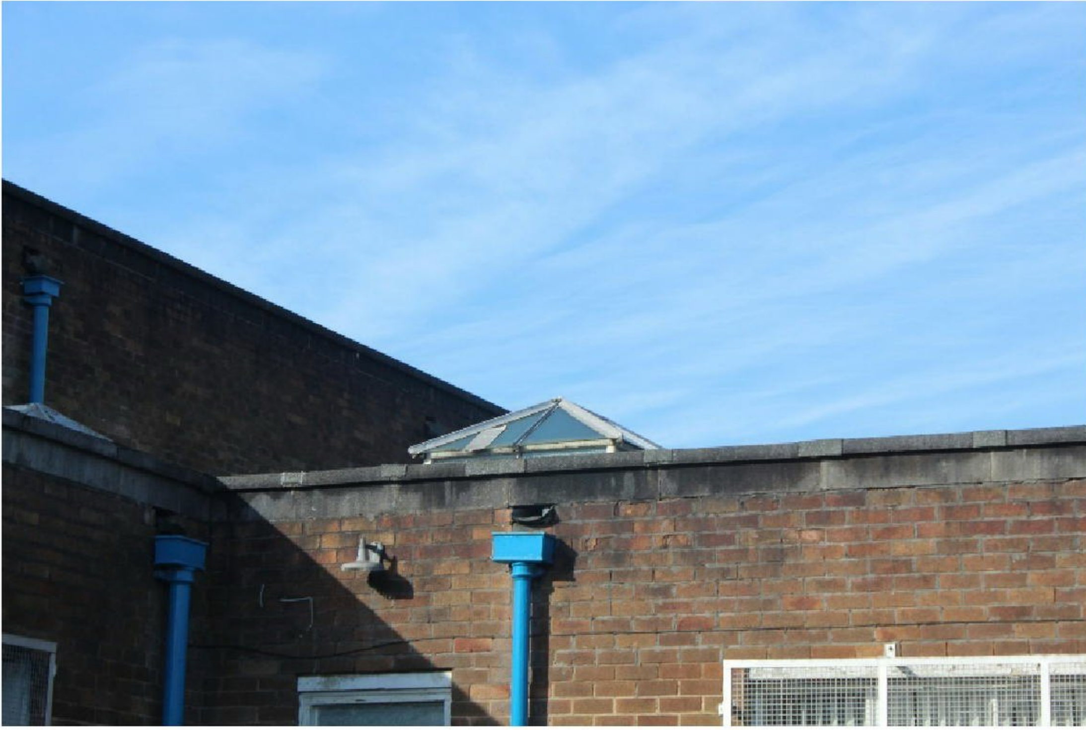
Glass roof lights in good condition
