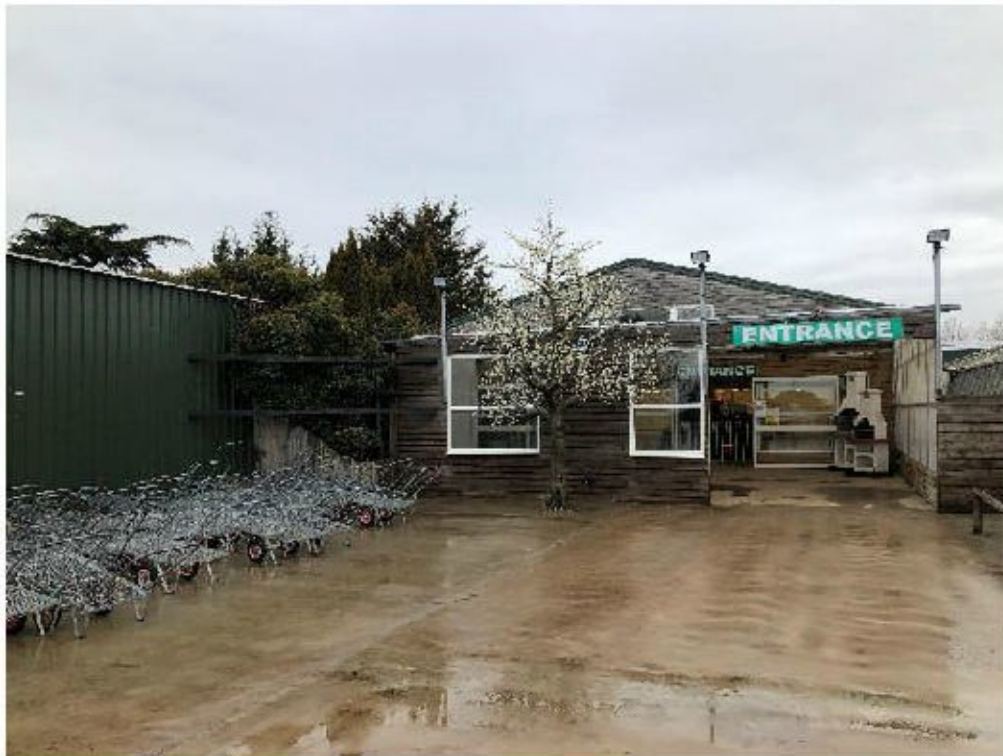
Photograph 15 Building reference M showing wooden panelling
