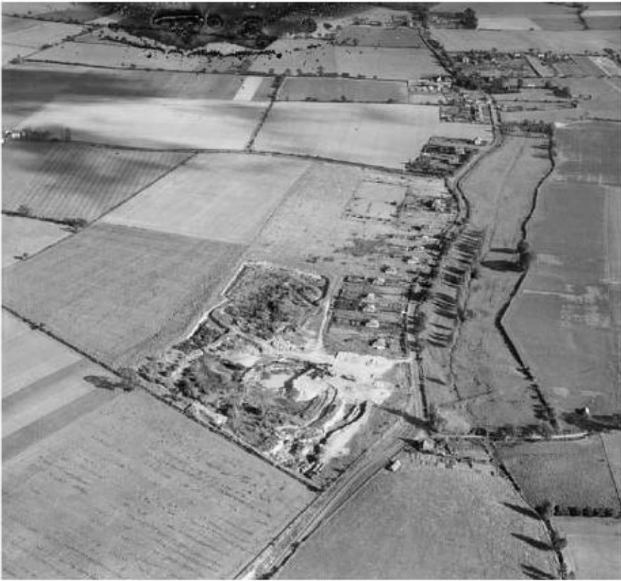
6. Aerial view of St Johns Road, Clacton-on-Sea, 1951 (Britain from Above)
