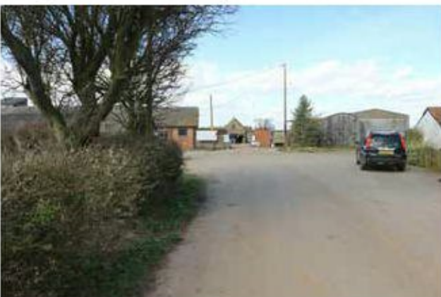
20 Farm buildings, Earl's Hall Farm, looking north from Earl's Hall Drive
