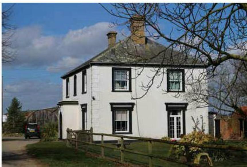
16 Earls Hall Lodge, south elevation
