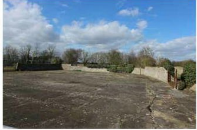
15 Hardstanding to the rear of Duchess Farm
