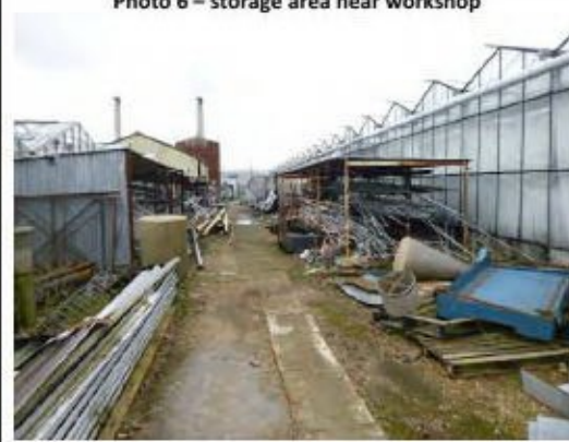
Photo 6 – storage area near workshop
