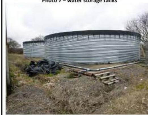
Photo 7 – water storage tanks
