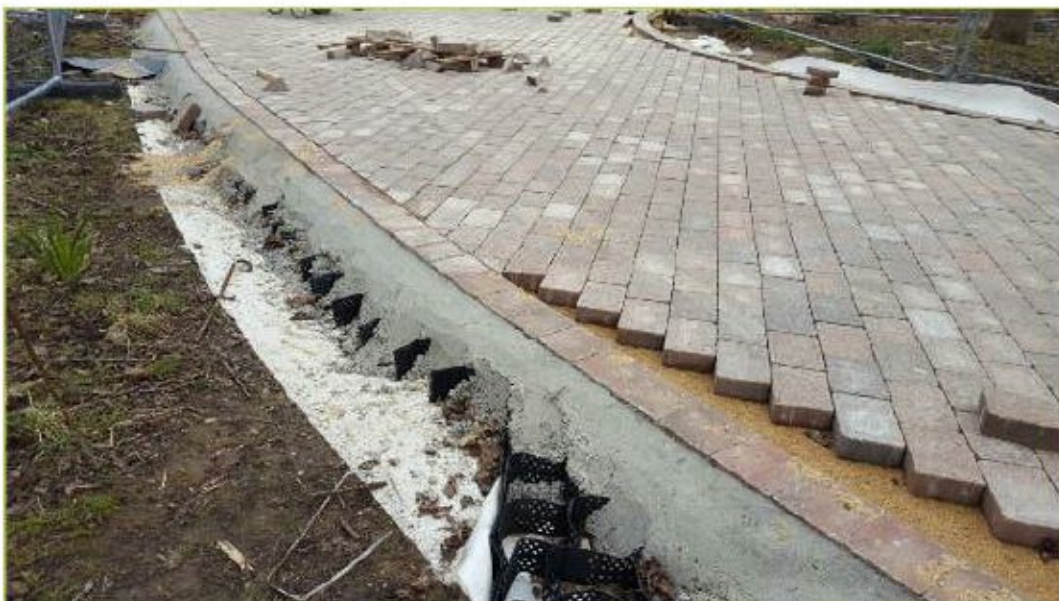
Photographs of 'Reduced-dig' 3D webbing system ground protection
