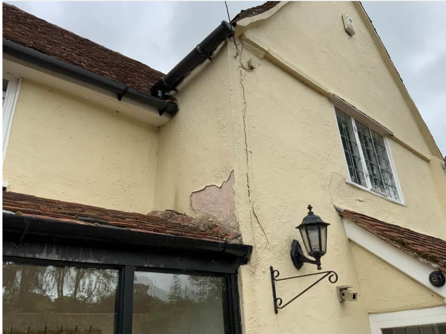
Figure 3 - Cracking to front
