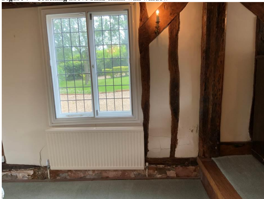
Figure 8 - Blown wall finish
