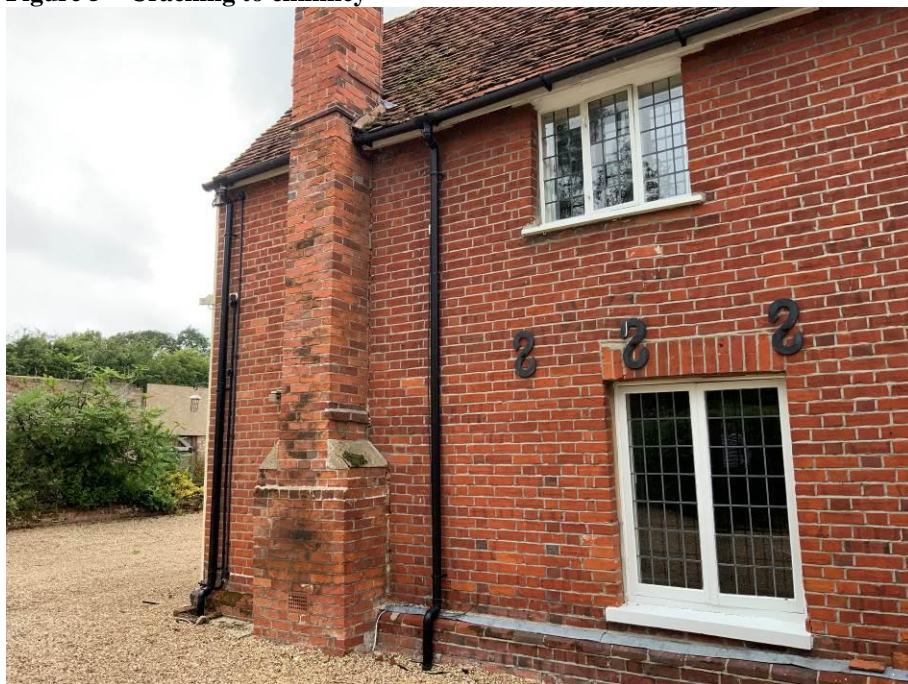
Figure 6 - Separation between chimney & wall
