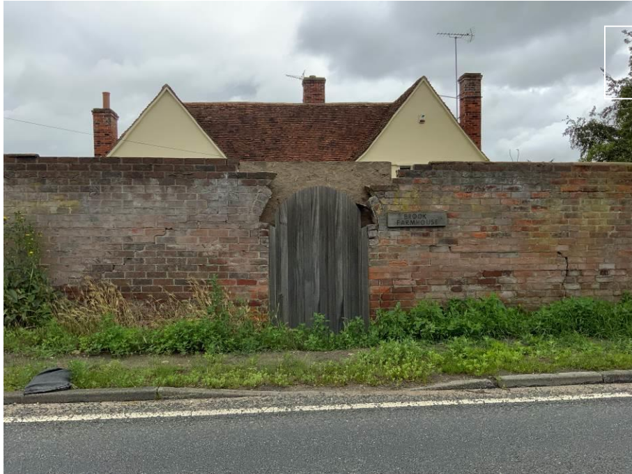
Figure 1 - Collapsed arch to boundary wall
