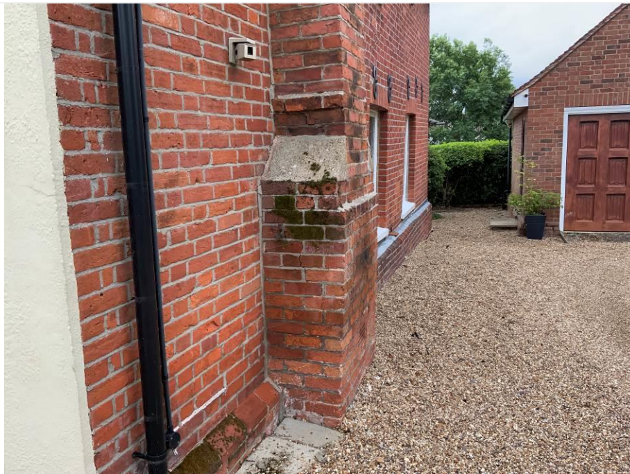
Figure 5 – Cracking to chimney
