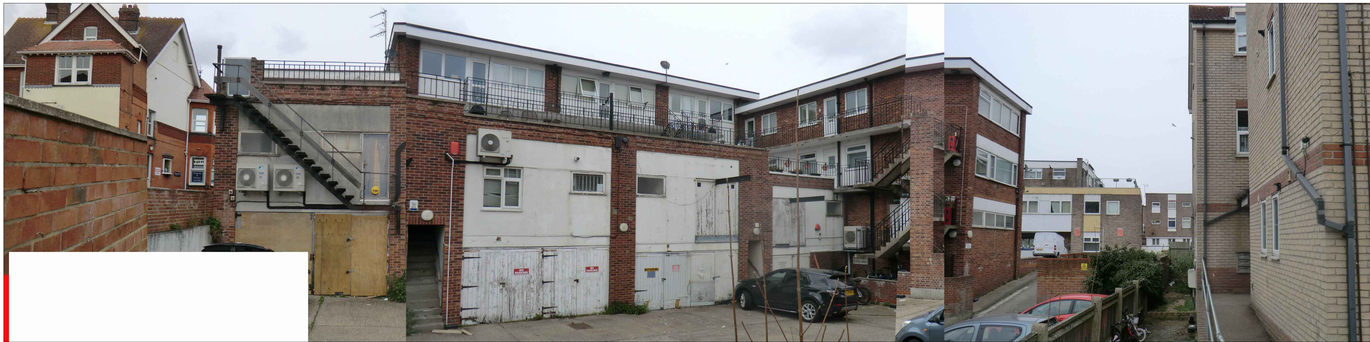
REAR OF STEELE HOUSE AS EXISTING
