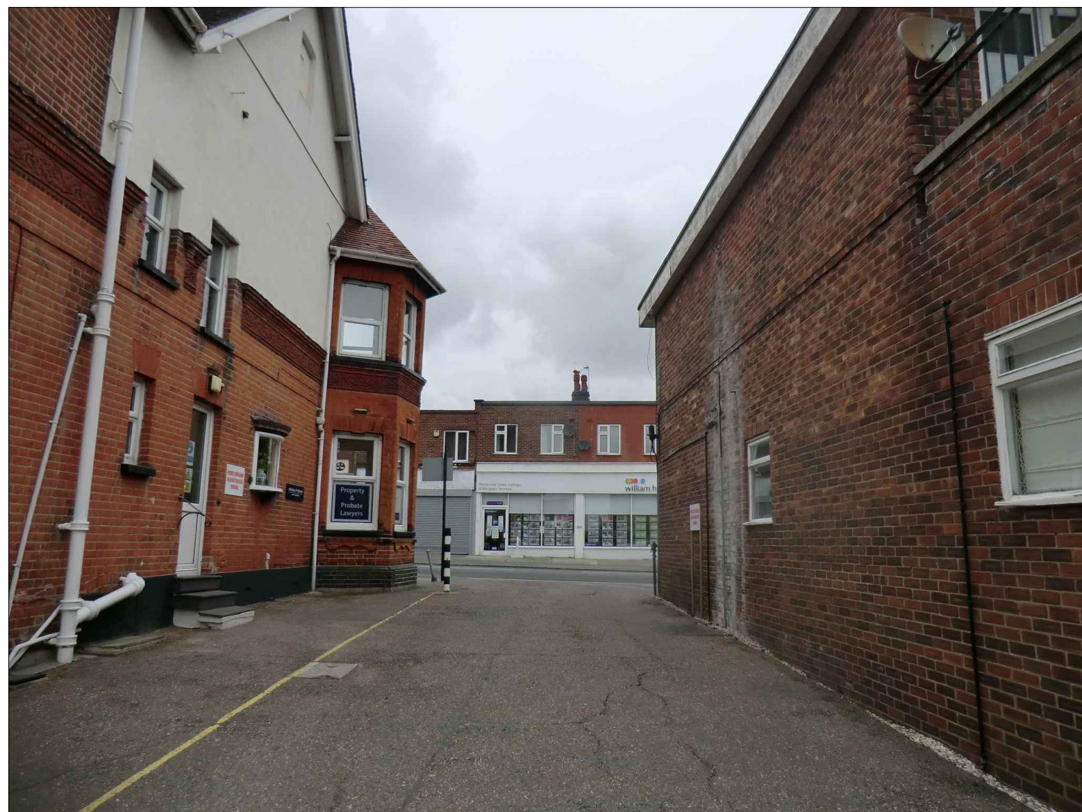
THE AREA TO THE WEST OF STEELE HOUSE AS EXISTING
