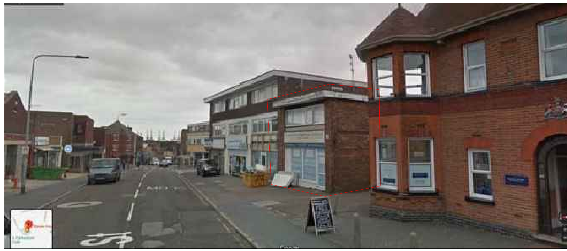
FRONT OF STEEL HOUSE AS EXISTING
