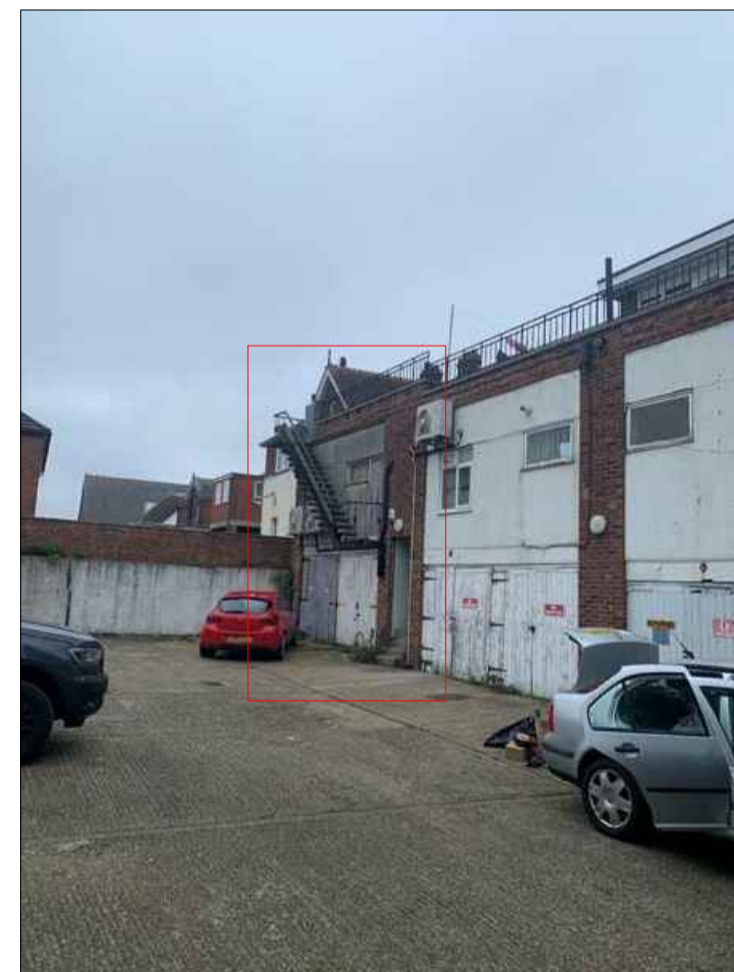
EXISTING REAR CAR PARK
