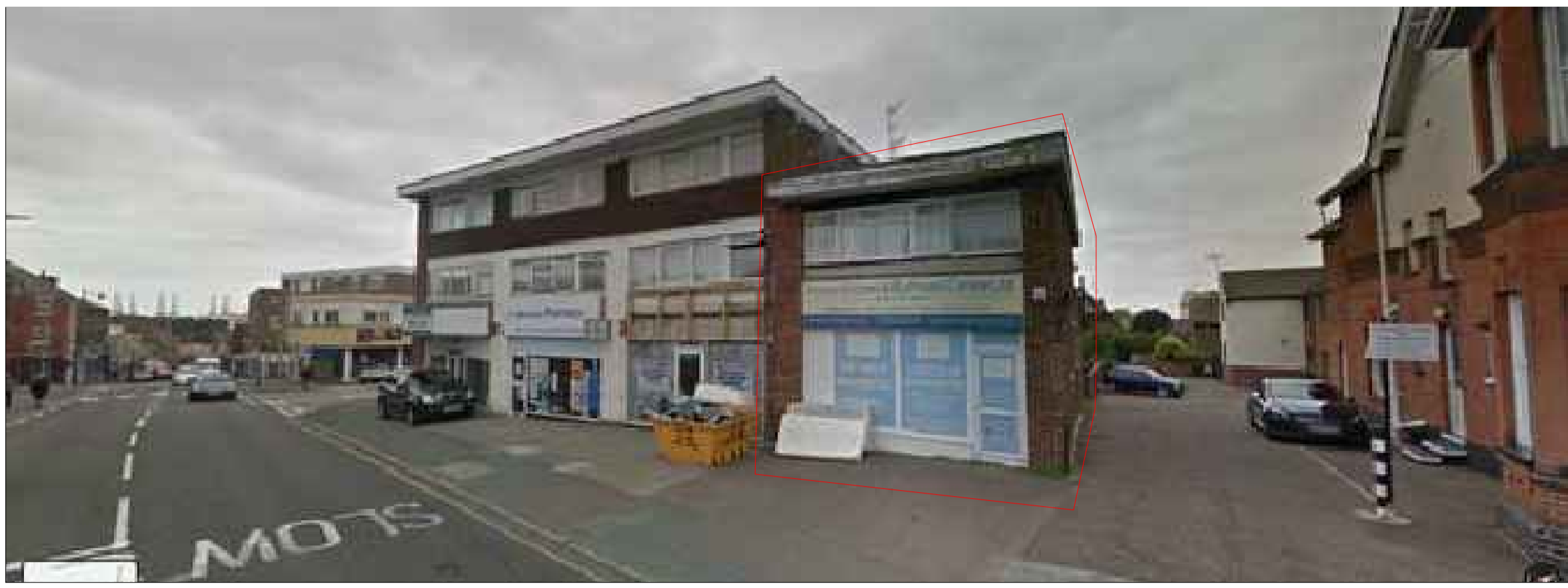
FRONT OF STEEL HOUSE AS EXISTING
