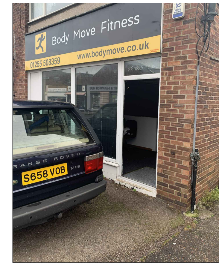
FRONT OF NO.5 STEELE HOUSE AS EXISTING
