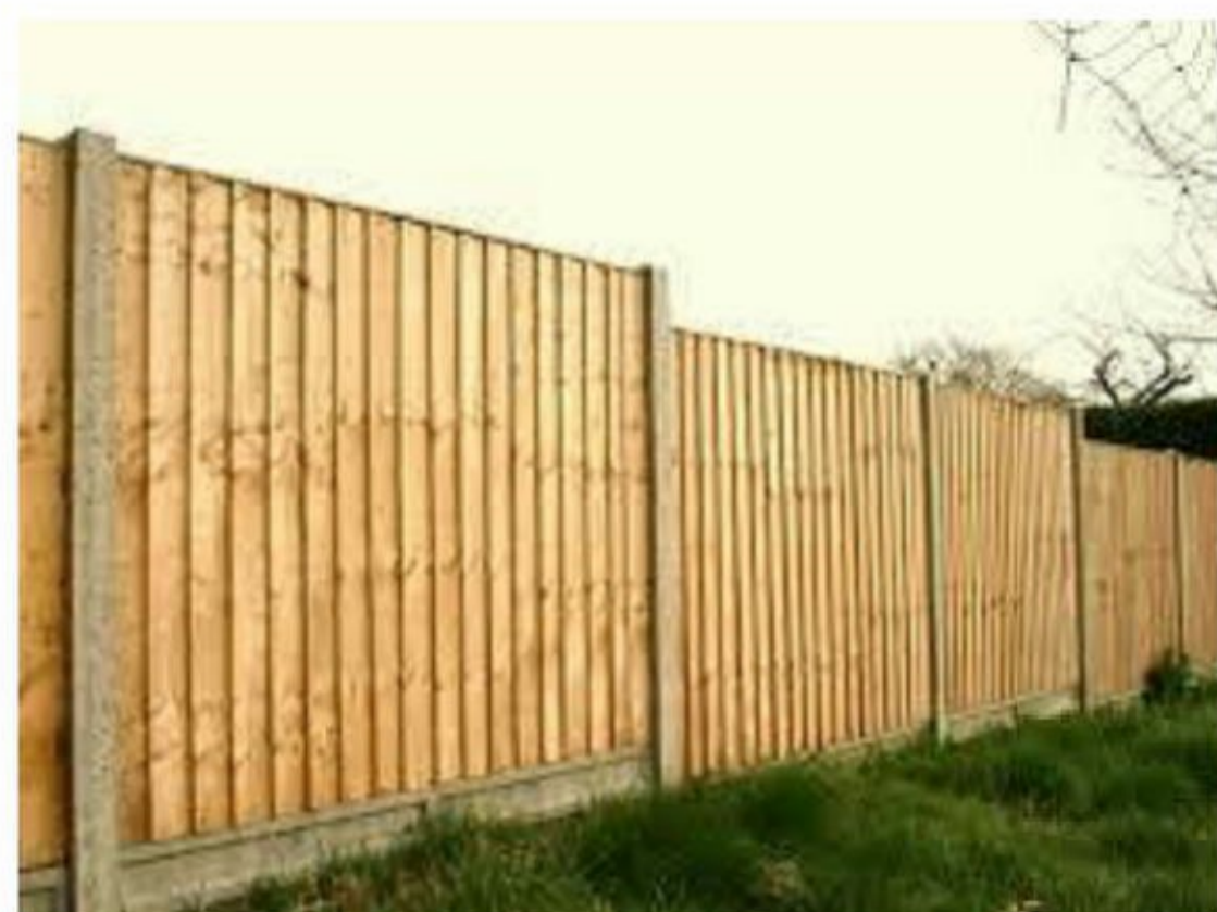
BOUNDARY TREATMENT FENCE TYPE 1 REAR GARDEN. 1.8M CLOSE BOARDED FENCING WITH CONCRETE POSTS AND GRAVEL BOARDS.
