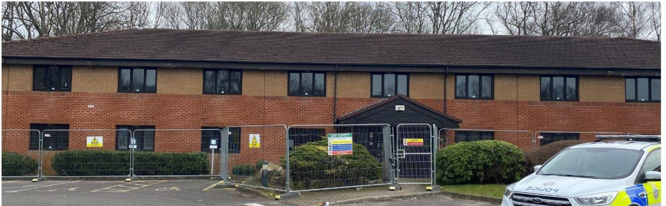
Photograph of the existing front elevation of the former Travelodge
