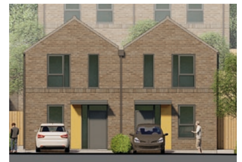
Plots 25 and 26 with grey multi facing brick and feature render panels to entrance doors.
