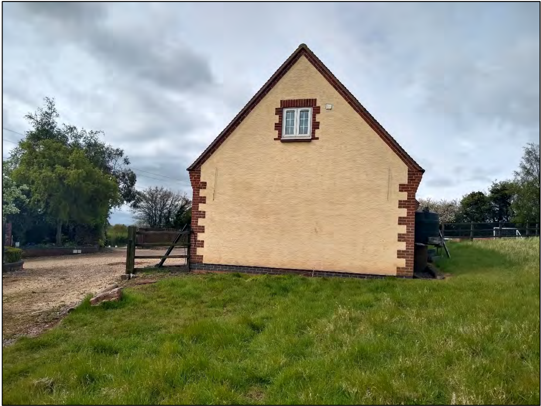
Photo 11: Northern elevation of the garage
