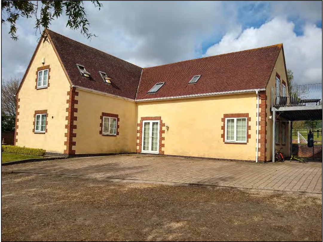
Photo 7: Eastern façade of main building
