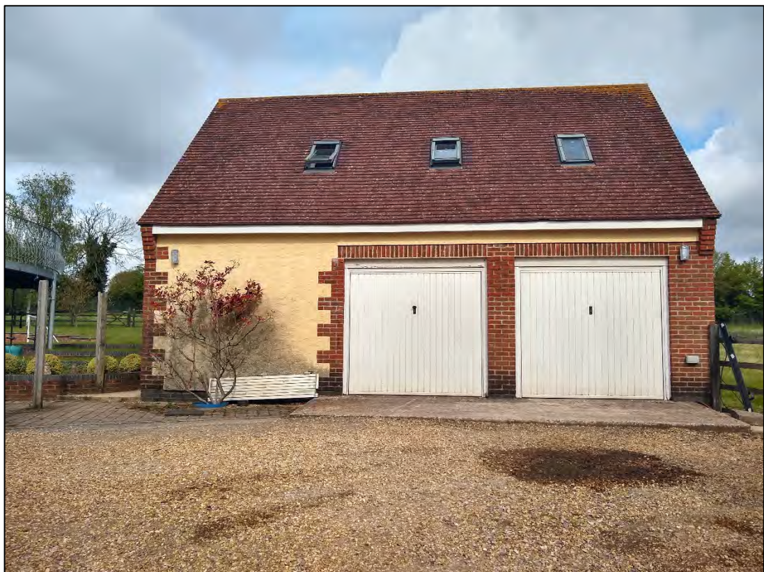
Photo 10: Eastern elevation of the garage
