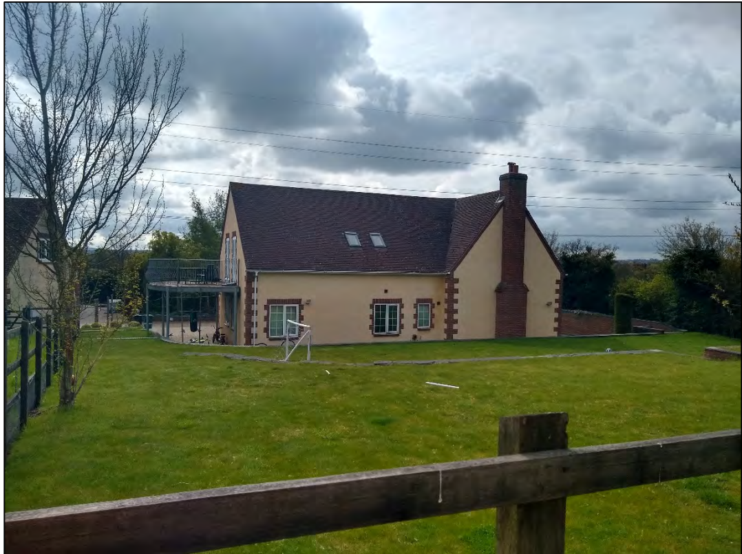
Photo 9: Western façade of main building
