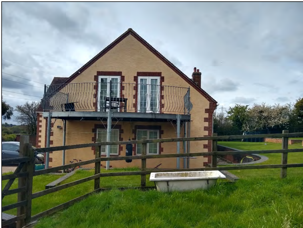
Photo 6: Northern façade of main building
