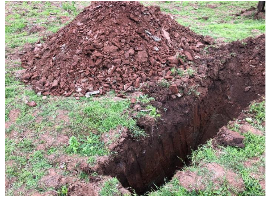
Photograph 3 – Displaying arisings (Mercia Mudstone Group) and trial pit of TP03 located, within the hummocked area in the centre of the site.
