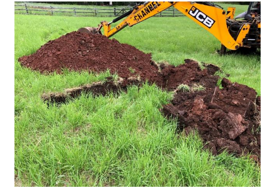
Photograph 5 – Displaying the arisings excavated from TP04, showing Topsoil (on the left) and the Mercia Mudstone Group (right).
