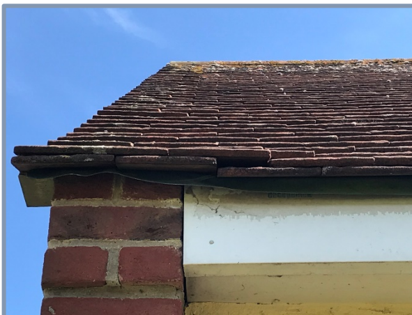
Photograph 4: Gaps under the tiles at the north-western corner of B2.
