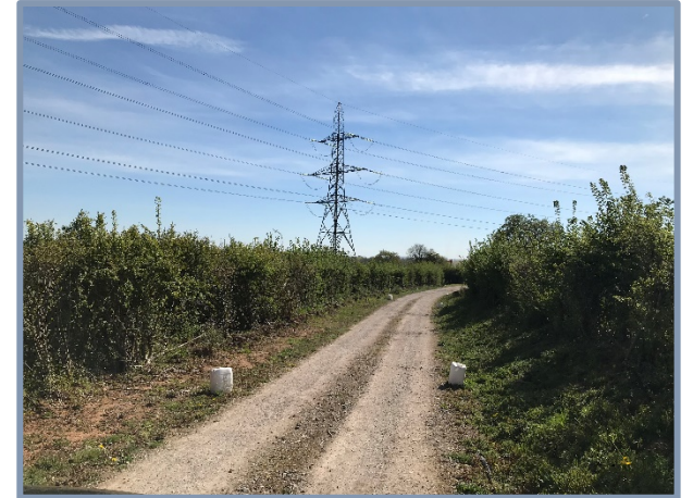
Photograph 13: View down the track with H7 on the left and H8 on the right.
