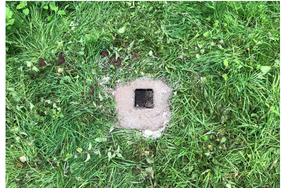
Photograph 6 – An example installation, taken from WS04.
