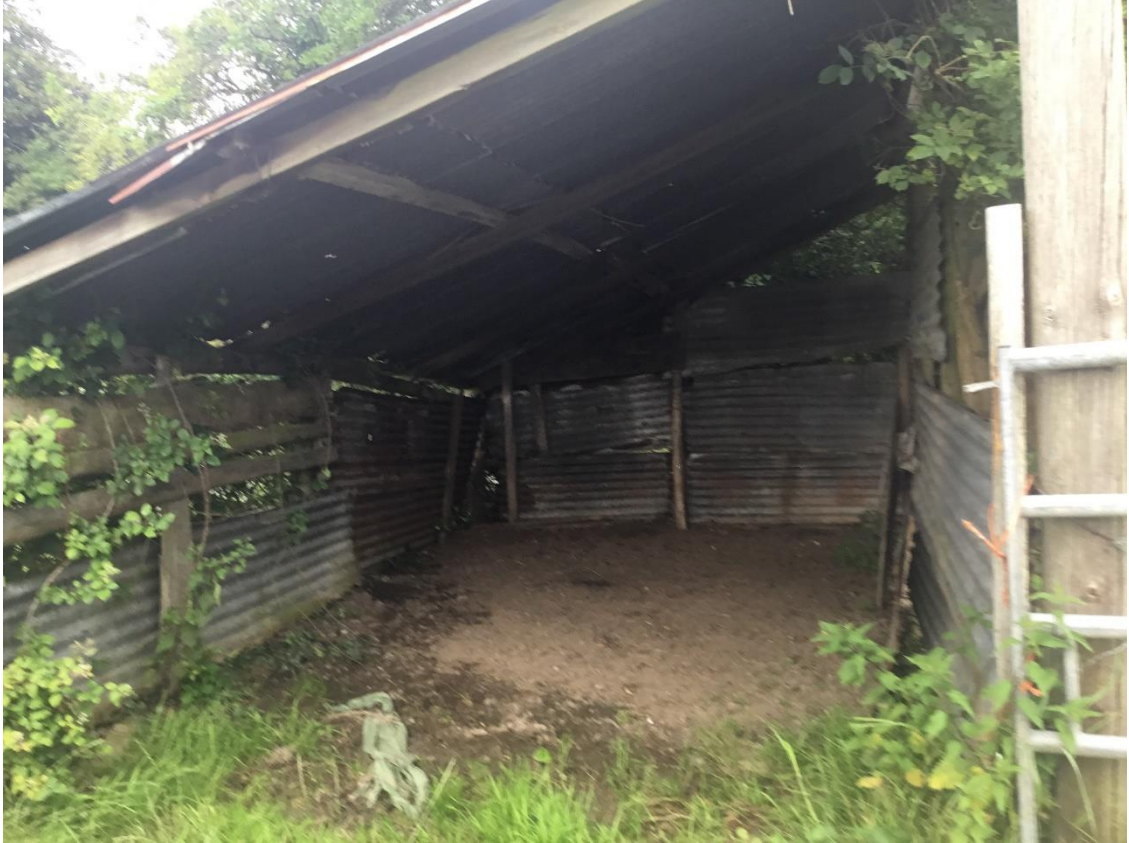
Figure 3: Timber framed barn at Ash Tree Farm
