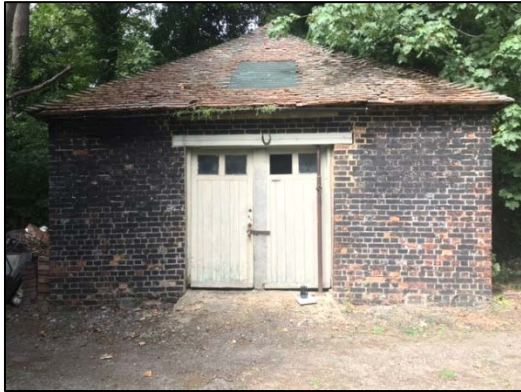
Photograph 4. The southern aspect of the stable with the double timber stable doors, show the gaps underneath the lifted roof tiles and the patch of missing tiles.
