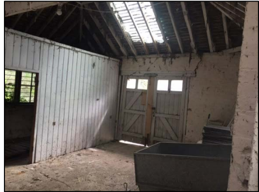
Photograph 6. Interior view of patch in the roof missing tiles and the timber double doors to the barn
