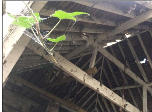
Photograph 7. Internal view of the timber framed roof of the stable block with no lining or insulation.
