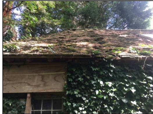
Photograph 5. Example patch of roof showing the gaps amongst the tiles and the vegetation cover.
