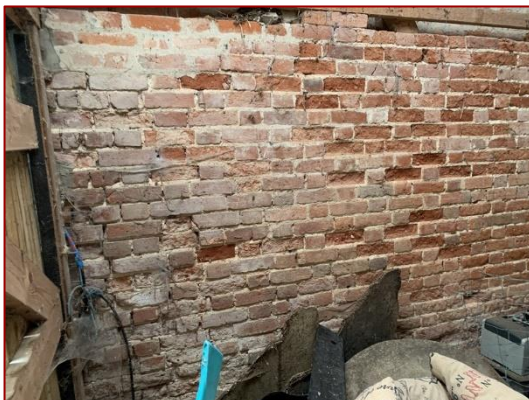
Photo 23: Internal view of Southern end of West Wing
