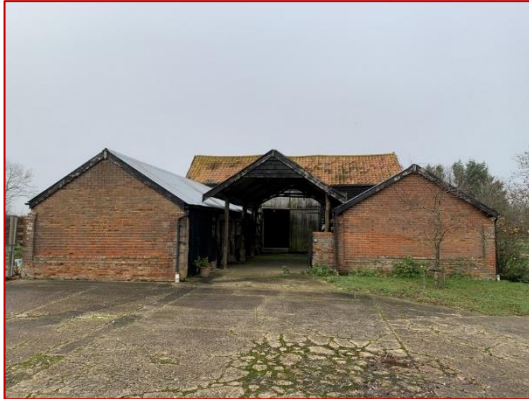
Photo 3: General view of South Elevation
