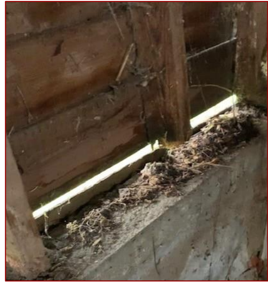
Photo 32: View of concrete encasement to timber wall plate
