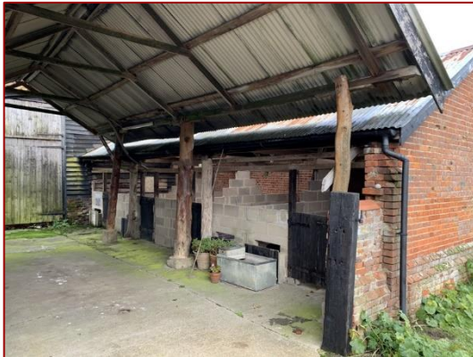
Photo 7: View of East Wing West Elevation
