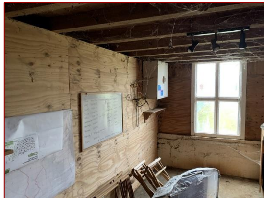
Photo 16: View of Western End ground floor of principal barn
