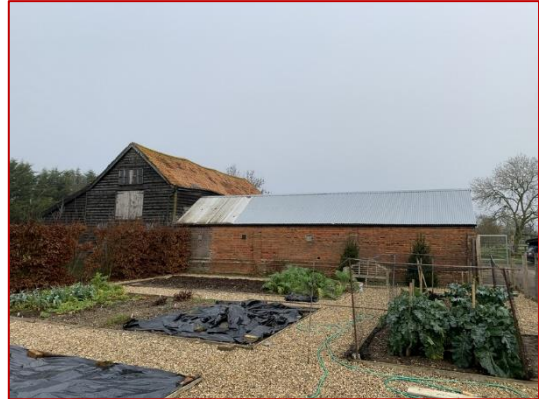
Photo 4: General view of West Elevation
