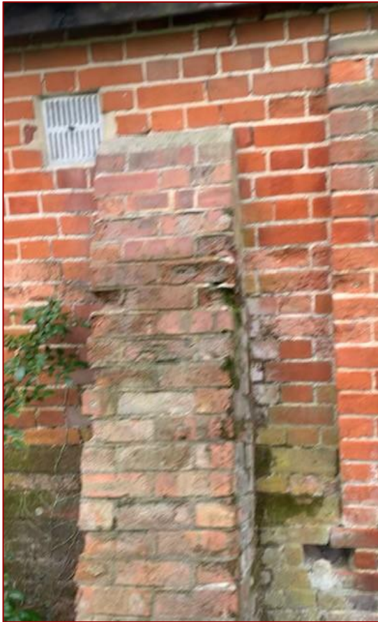
Photo 35: View of buttress to east elevation of east wing.
