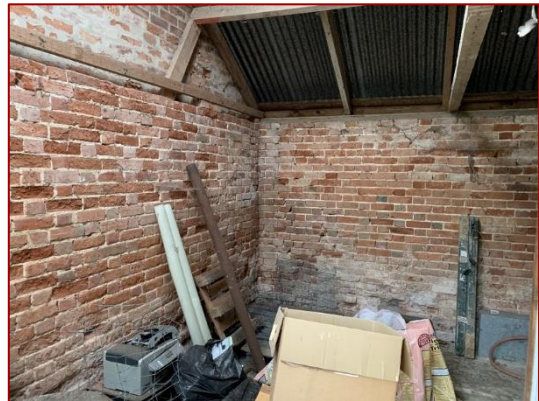
Photo 22: Internal view to Southern end of West Wing
