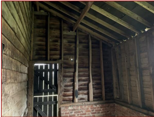
Photo 19: Internal view of northern annex
