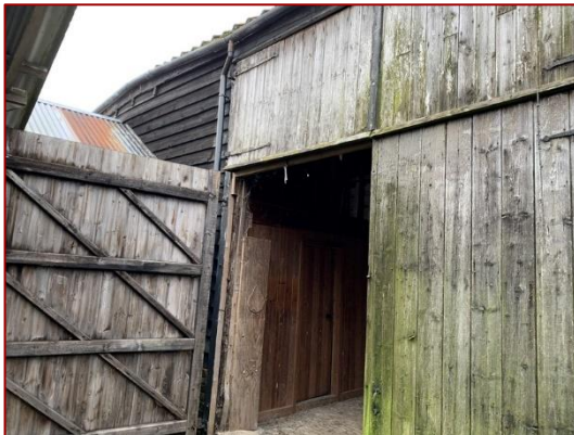
Photo 9: View of Main Barn South Elevation
