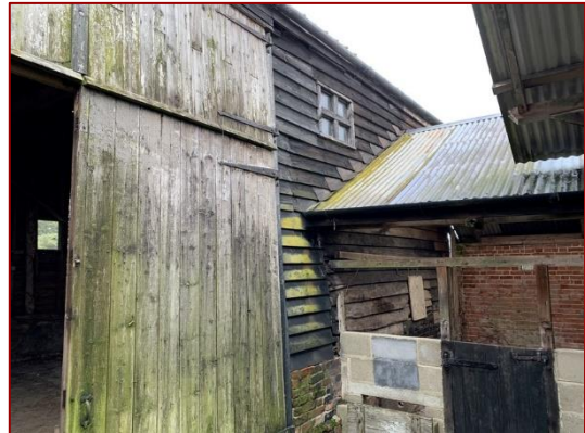
Photo 8: View of Main Barn South Elevation
