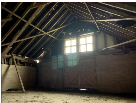
Photo 17: View of first floor at the Western end of principal barn
