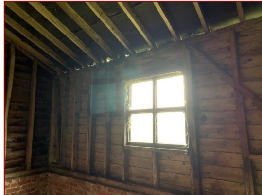
Photo 20: Internal view of northern annex
