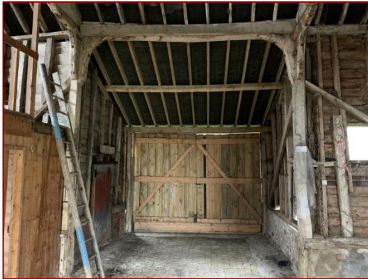
Photo 13: General internal view looking towards Northern porch
