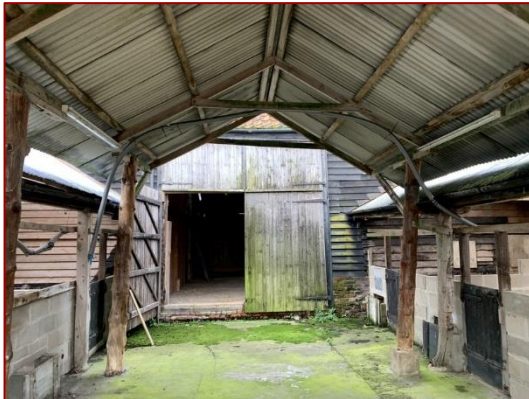
Photo 5: View of East and West Wing
