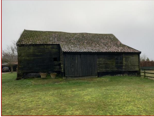
Photo 1: General view of North Elevation
