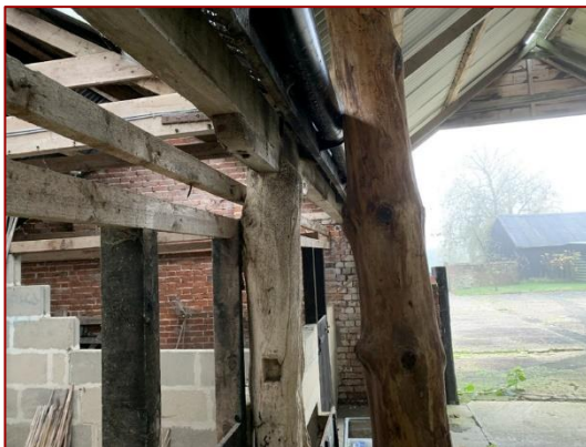
Photo 29: General view of post supporting roof structure to wings.
