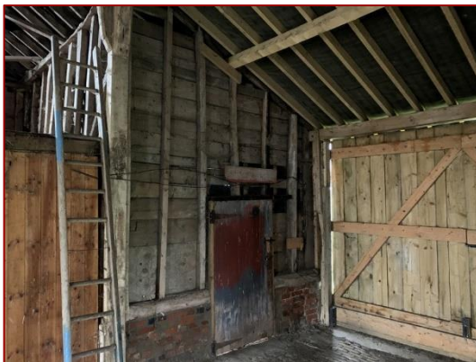
Photo 15: View of West Elevation of Northern porch
