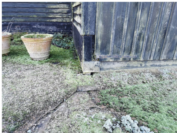
Hardstanding adjacent to the northern aspect of the complex
