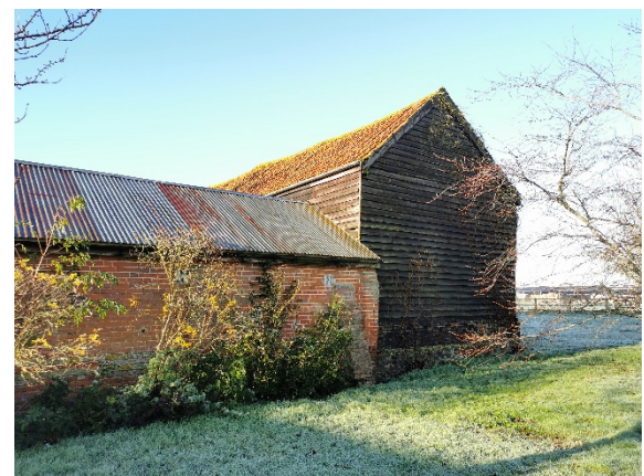
Eastern aspect of the complex
