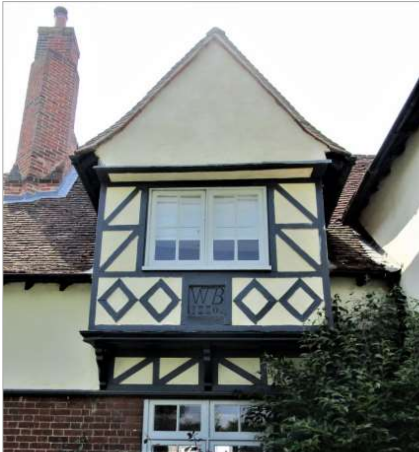
Fig. 7: Gabled oriel bay added to the hall range in 1880, the initials WTB standing for Walter Thomas Brown of Brent Eleigh Hall
