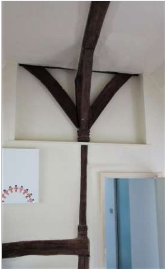
Fig. 2: Crown post in hall range
