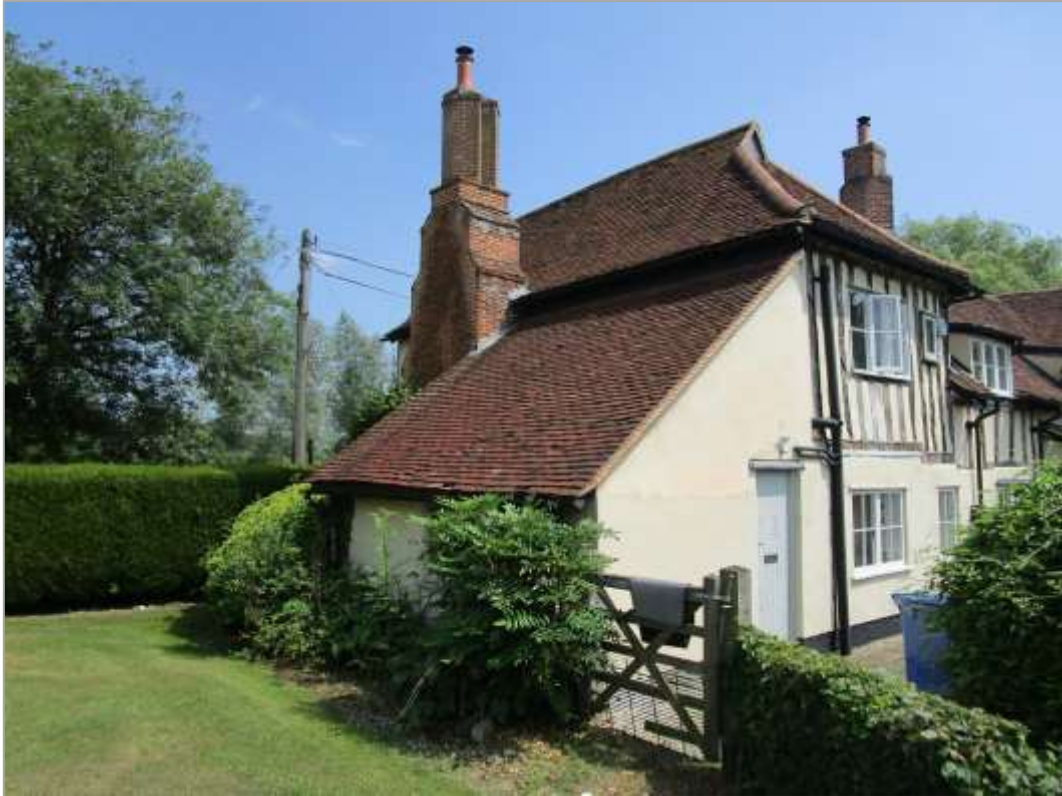
Fig. 12: The C20 lean-to addition from the NE. Its E elevation is aligned with the E elevation of the parlour range and is rendered. The N return elevation is also rendered, as far as the window (concealed by a shrub in this photo), and thereafter is of painted brick.
