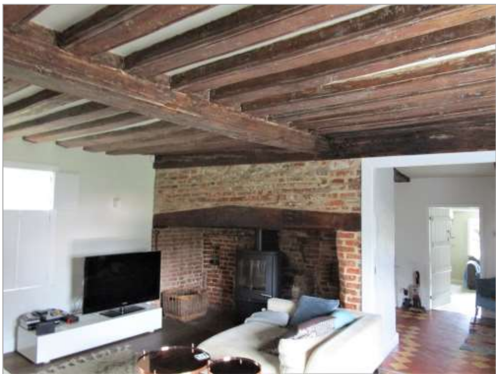
Fig. 3: Inserted C16 stack and floor in hall range
