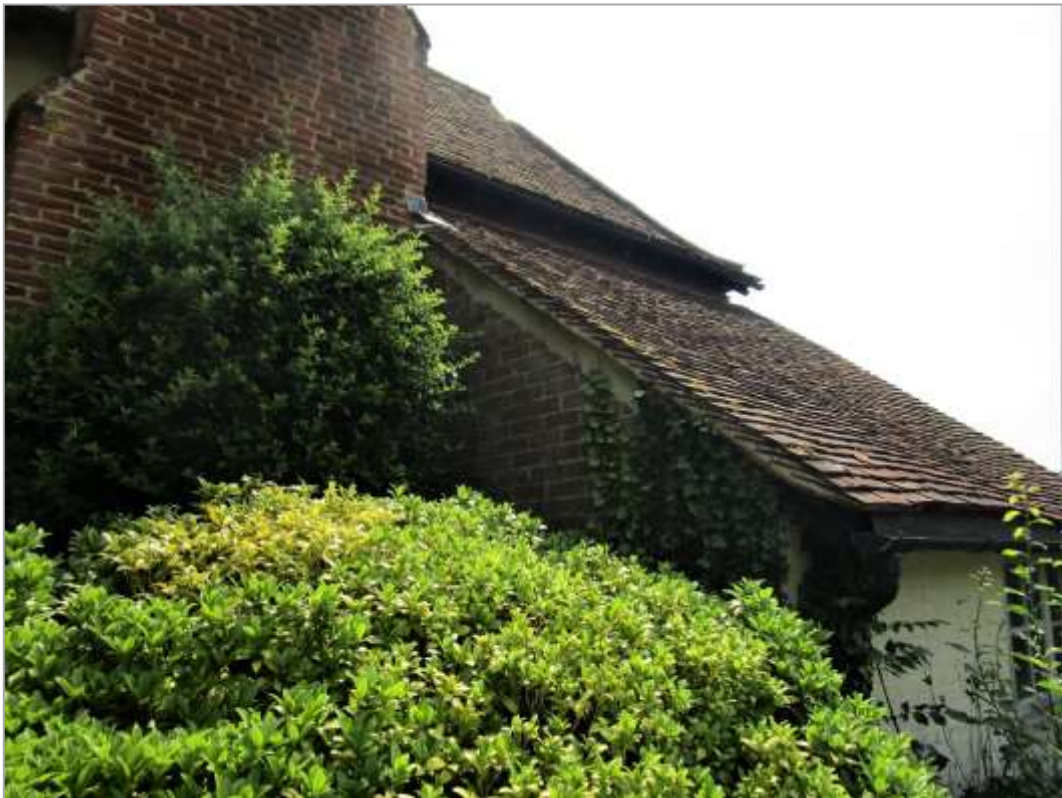
Fig. 13: The upper part of the S elevation of the lean-to, abutting the C16 stack and of unpainted red brick laid in stretcher bond.
