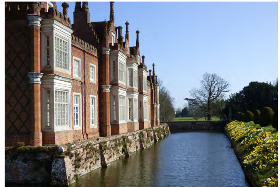
Helmingham Hall - the South-West Elevation
