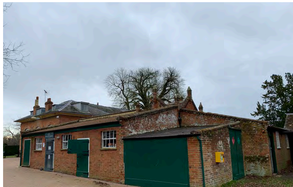
The shop – exterior view on arrival. The shop and ticket sales are accessed via the grey door
