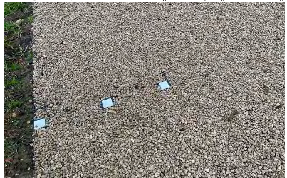
Stone clippings within retention grid: to be used for accessible parking spaces (grey granite chips proposed to match main drives).
