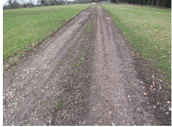
Photo 2: Existing mud track / bare earth
