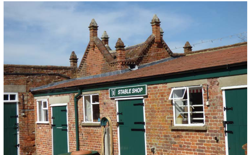
The 'enveloped' pavilion in the Stable Yard
