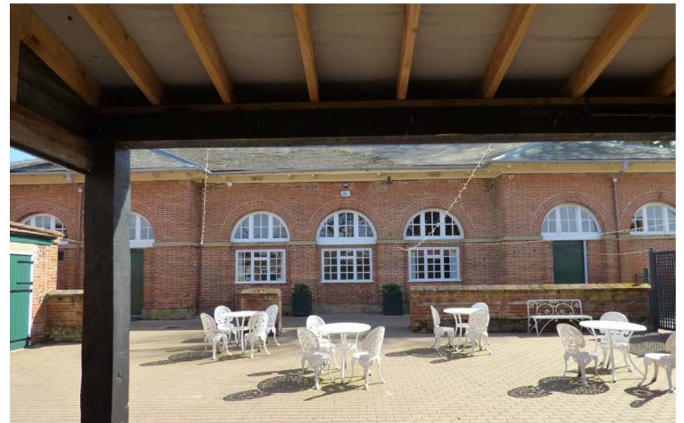
Stable Yard - view of Stables: note the central bay originally had a door (now blocked). The three ground floor windows serve the current tea room.
