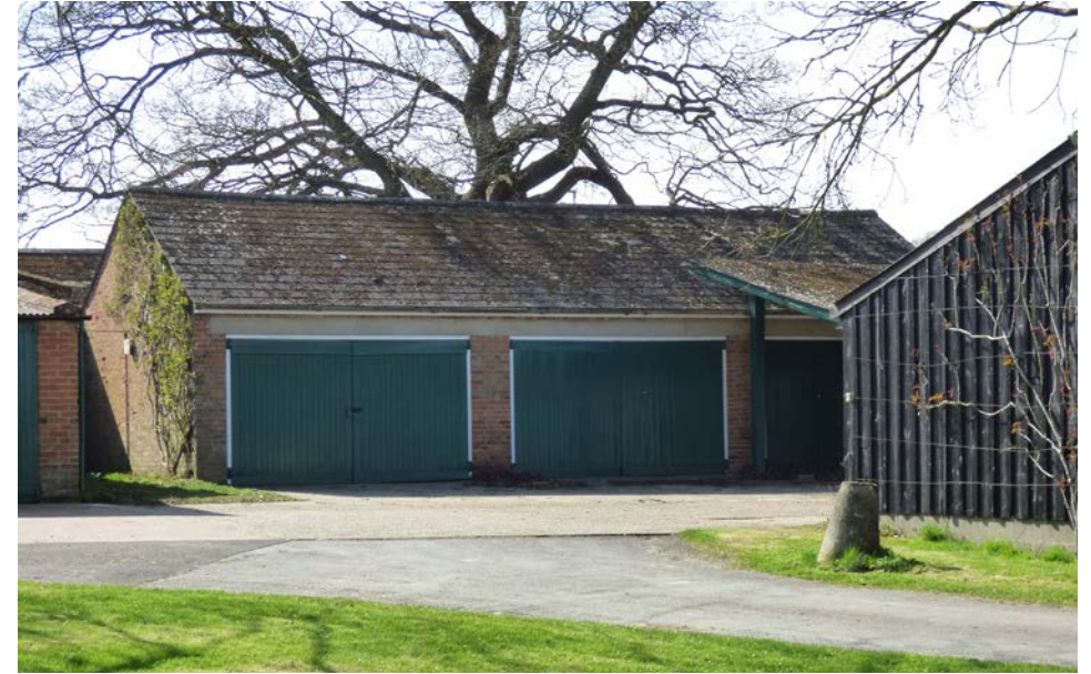
Garage/Store - a building which could potentially be repurposed as the shop or visitor reception
