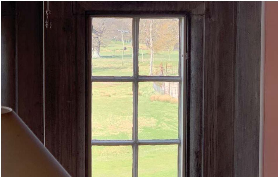
View from the first floor room bedroom window at the west corner of the house
