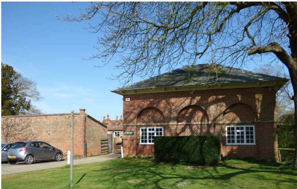
Stables - South-west elevation (viewed from the Hall)
