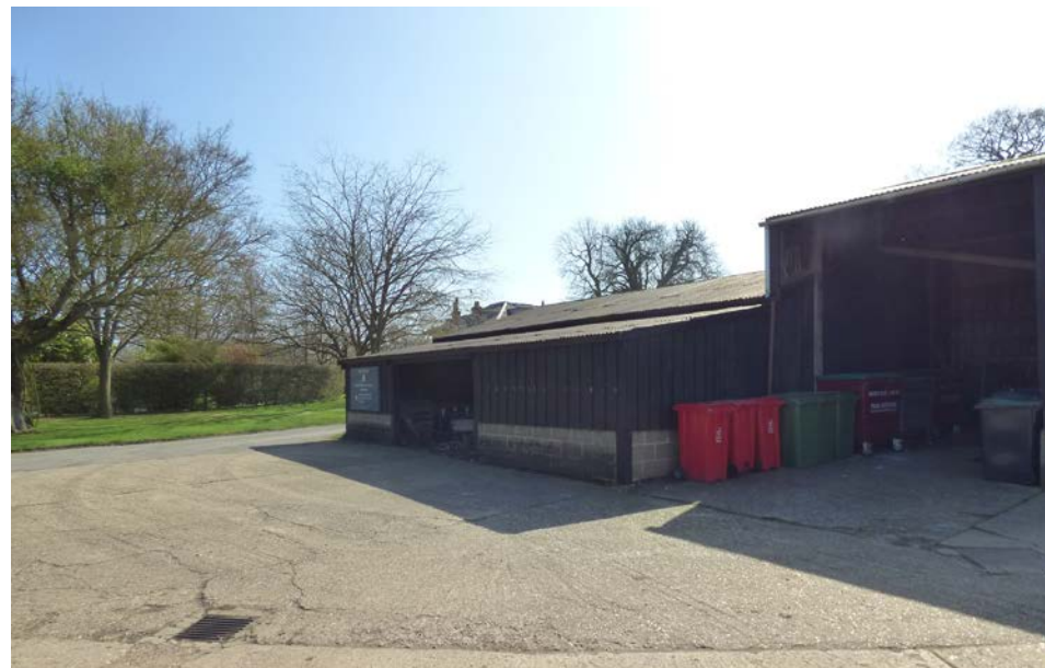
Garage, wood store and bin store from the North (this building assumed to be demolished)
