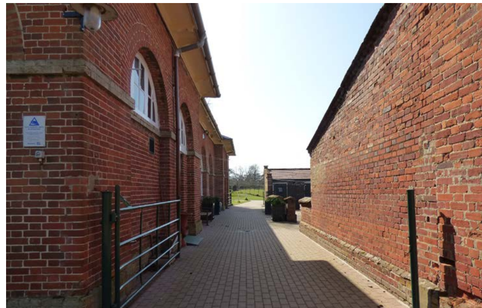
View along North-East elevation of stables, through the yard
