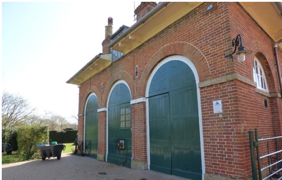
North-East elevation of Stables
