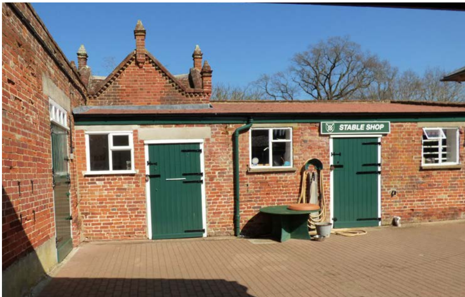
North corner of Stable Yard: is this the enveloped pavilion apparent on Isaac Ware's map of 1803?
