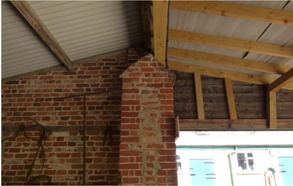
North-west side of Stable Yard: remnant of former yard wall?
