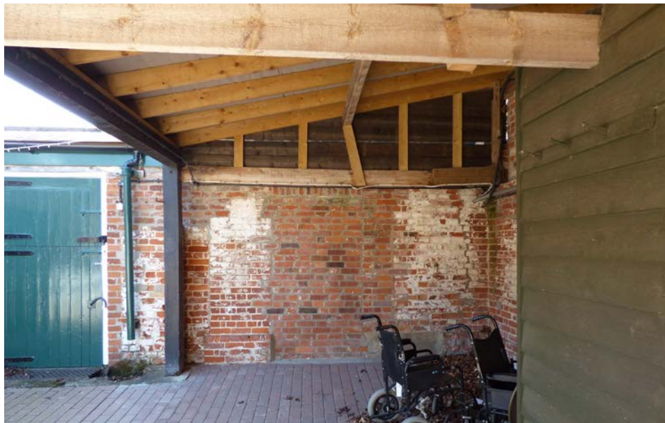
Stable Yard: view to North-West corner showing inserted roof potentially to be removed. Note also the blocked doorway and possible remnants of the North East 'pavilion' apparent on the Isaac Ware map of 1803
