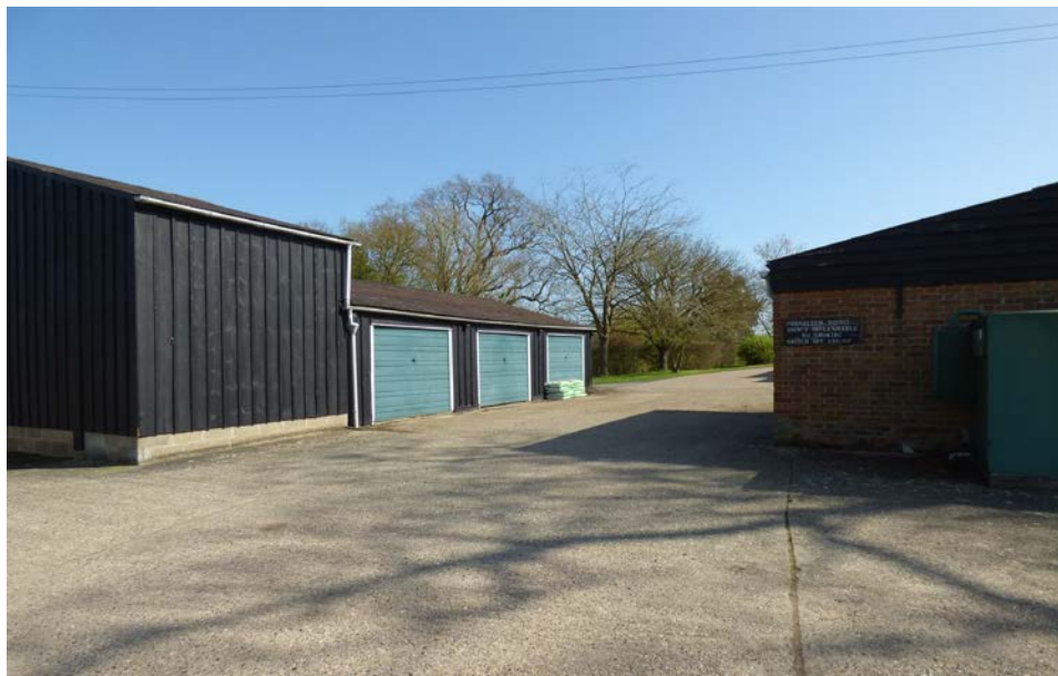
Garage yard from the North west
