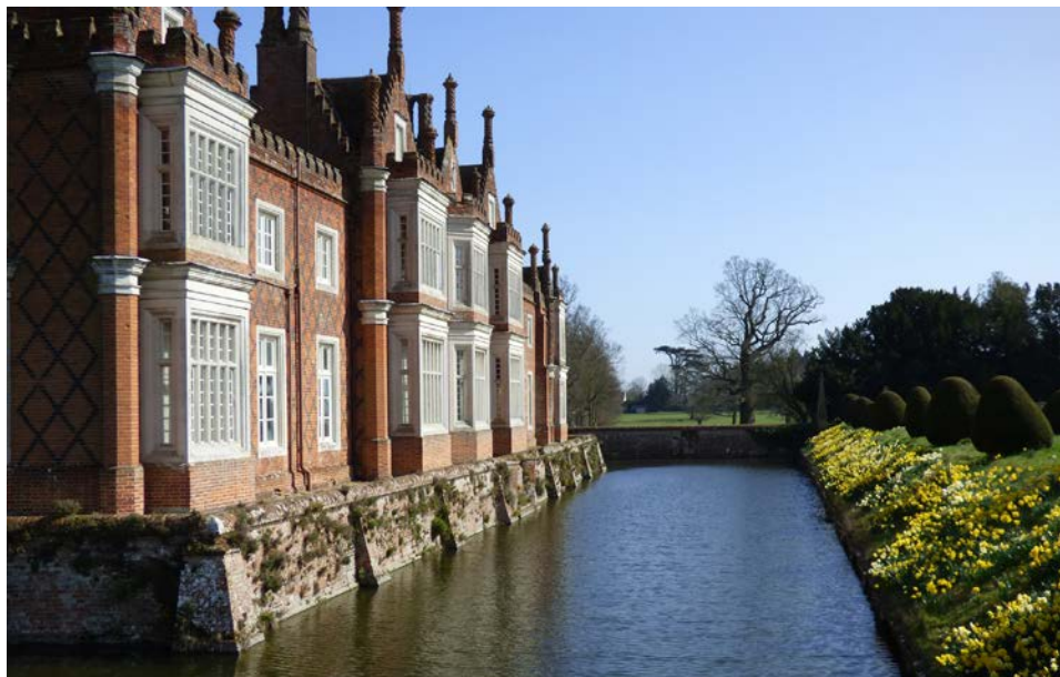
View of the South-West elevation of the Hall, looking onto the main gardens
