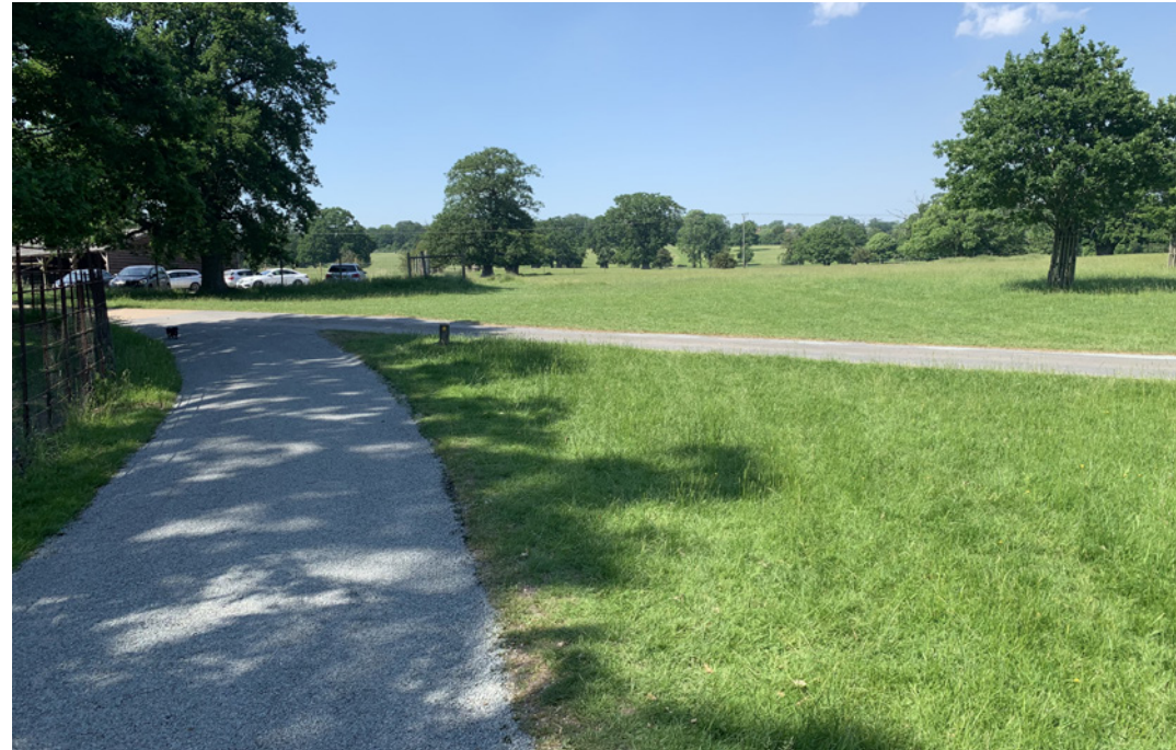
Surfaced access to car park to be finished with grey granite chippings and no kerbs to match existing drive, as illustrated
