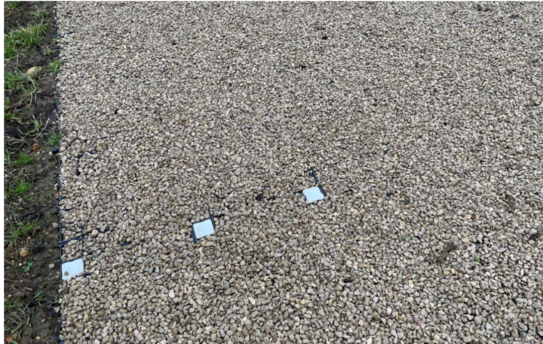
Grey granite chippings 6-12mm diameter proposed for areas of hard standing, within gravel retention grid for accessible parking and route to coach parking bays, as illustrated
