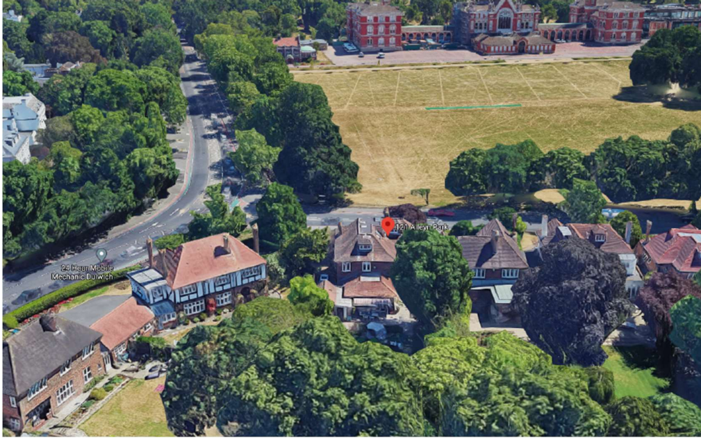
02 Image: Rear Ariel View of the Back of Application Site Source: Google Maps
