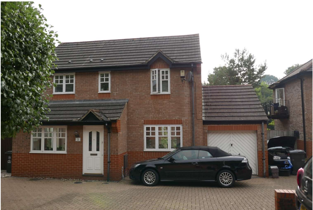
Figure 1 - Front of 3 Anchor Close
