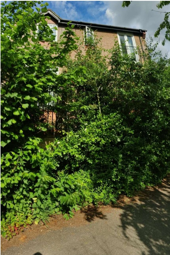
Figure 4 – Path View, looking East
