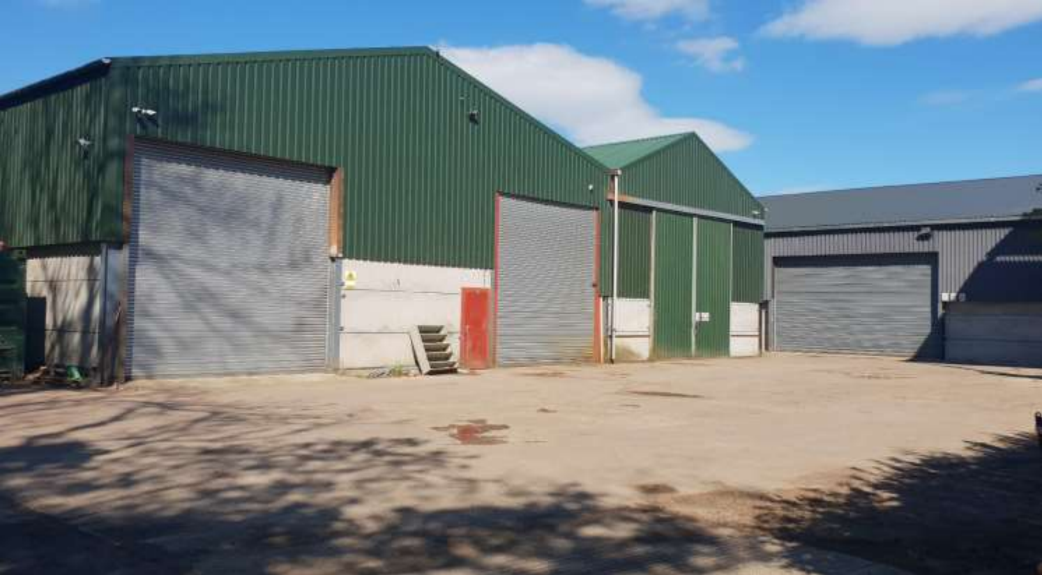
Photograph 3: Yard to the east of the main building, adjacent to proposed development site
