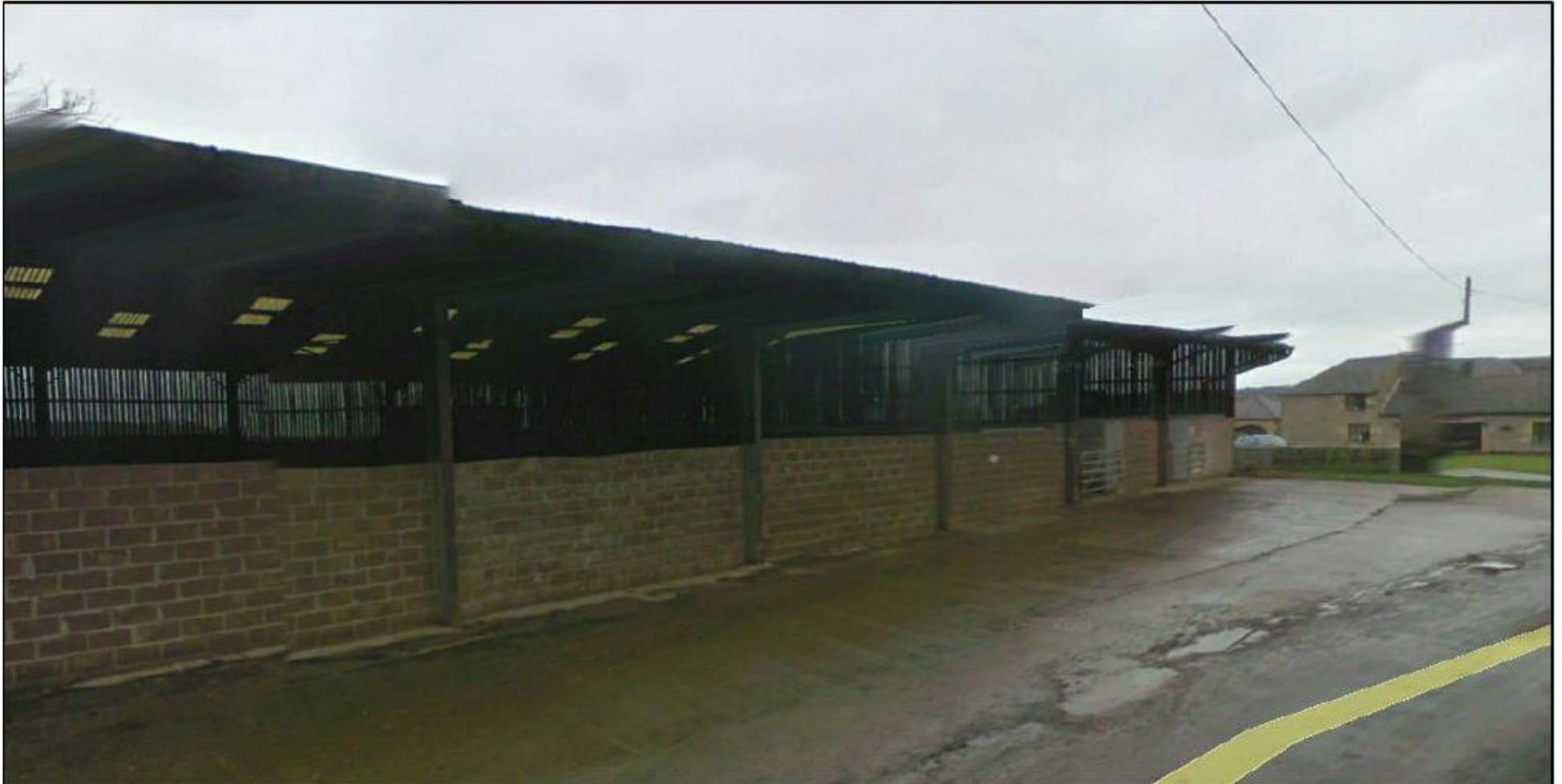
Building on site
