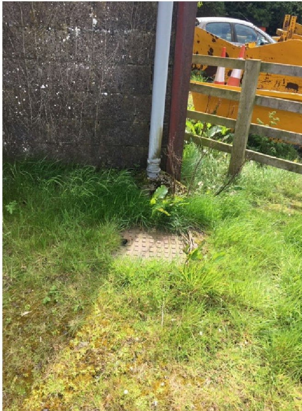
Photograph Showing RWP in North West Corner Discharging into Sewer
