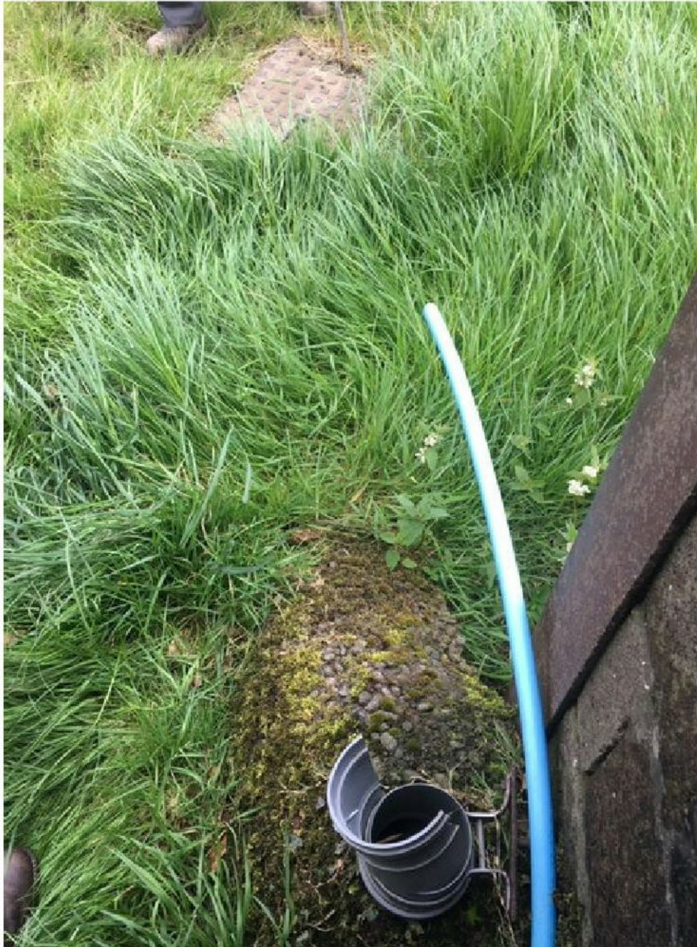
Photograph Showing RWP in North East Corner Discharging into Sewer
