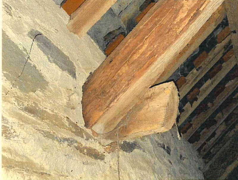
Photograph 12 – Original timber collar tie at eaves level cut off.
