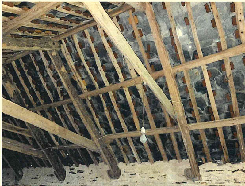
Photograph 13 – Common rafters glued to foam blocks and purlins.
