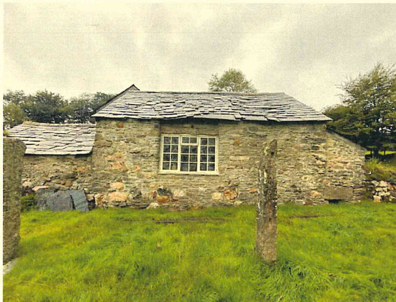
Photograph 24 – Rear elevation at western end of barn.
