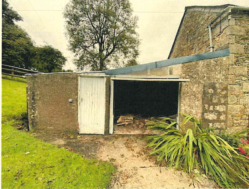
Photograph 5 – Front garage door opening and single door opening into plant room
