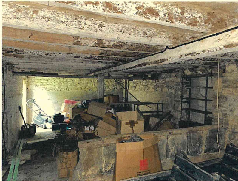
Photograph 7 – Timber floor joists to first floor of original barn.
