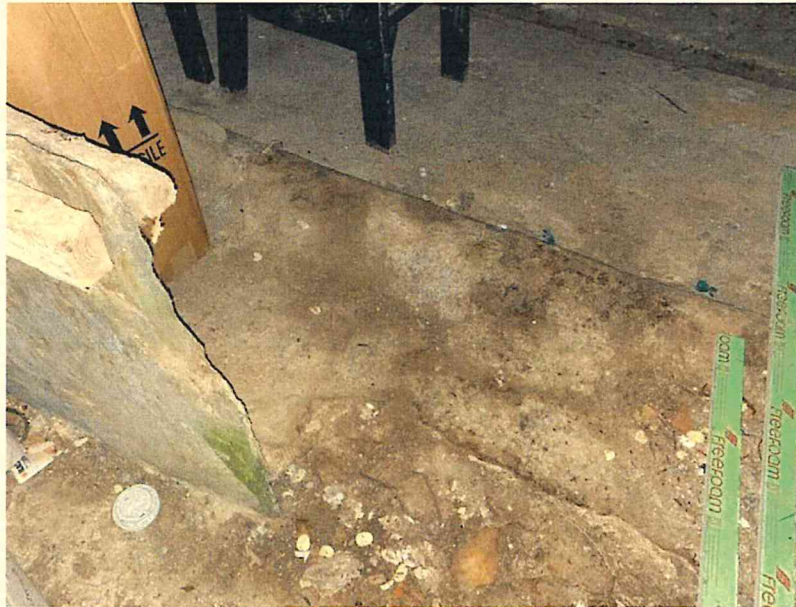
Photograph 10 – Example of ground floor construction..
