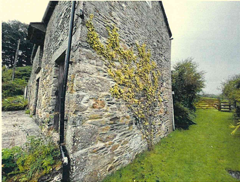
Photograph 4 – Later cement based pointing and foliage growth again gable.
