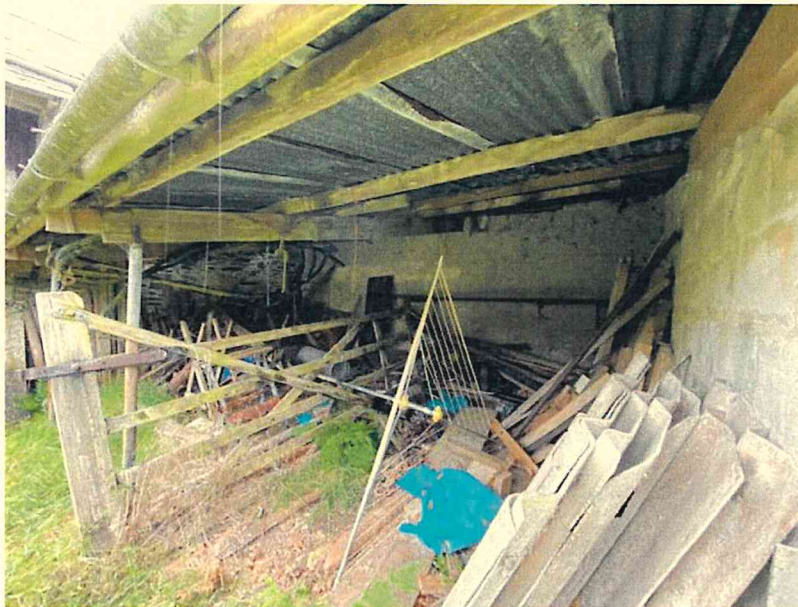
Photograph 16 – Open fronted section of roof structure at rear.
