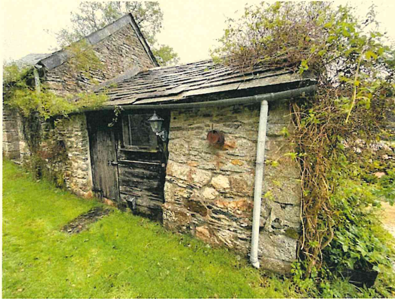
Photograph 21 – Front flank wall of eastern section of barn II.
