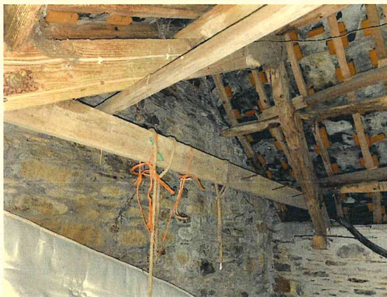
Photograph 26 - Truss structure to eastern end of barn.
