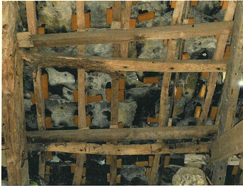
Photograph 27 – Purlins with common rafters and later foam pad fixings.
