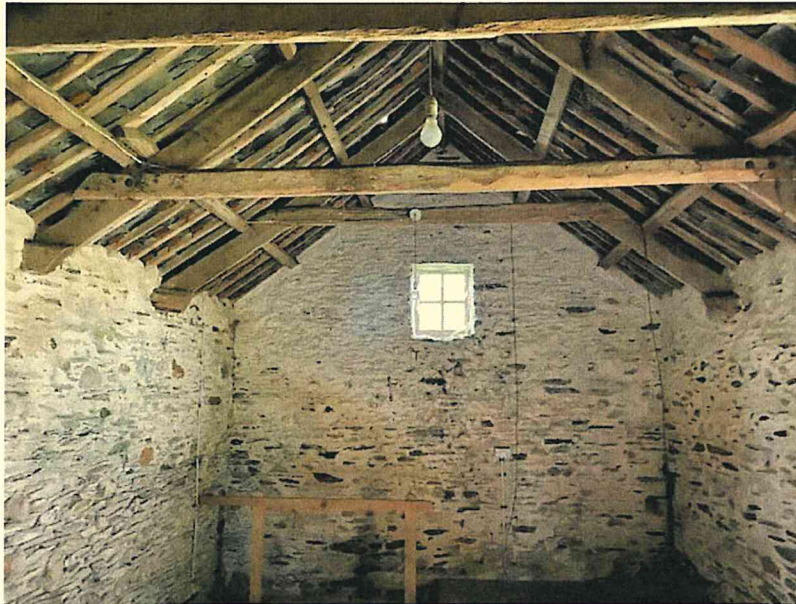
Photograph 11 – Raised A frame truss and purlin roof structure.
