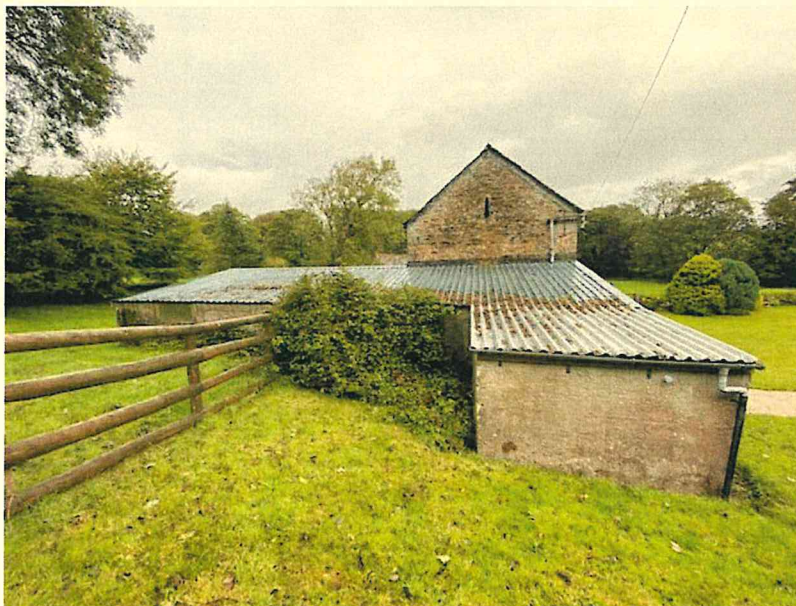
Photograph 6 – Side elevations of later concrete blockwork extensions.
