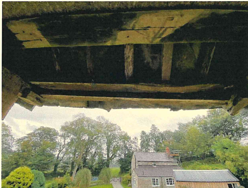
Photograph 14 – Underside of hayloft canopy roof structure.
