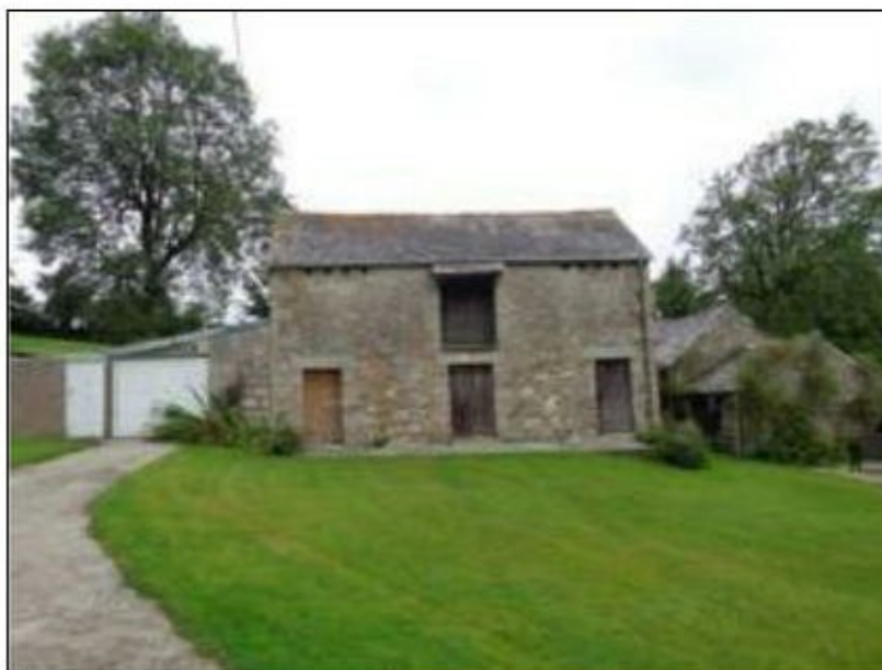
Figure 1. Barns viewed from the east
