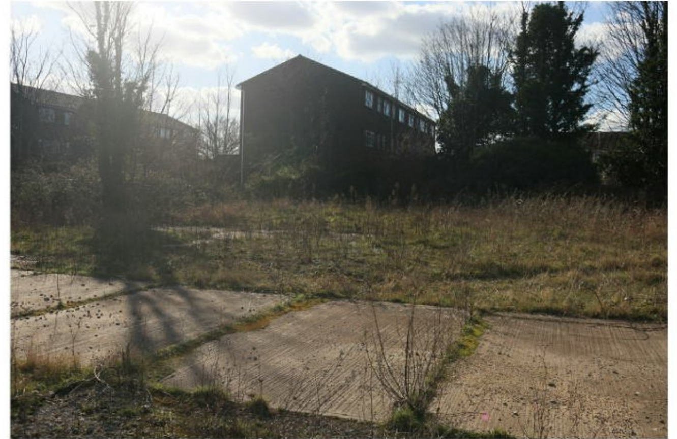
3 Storey Flats on Maple Close
