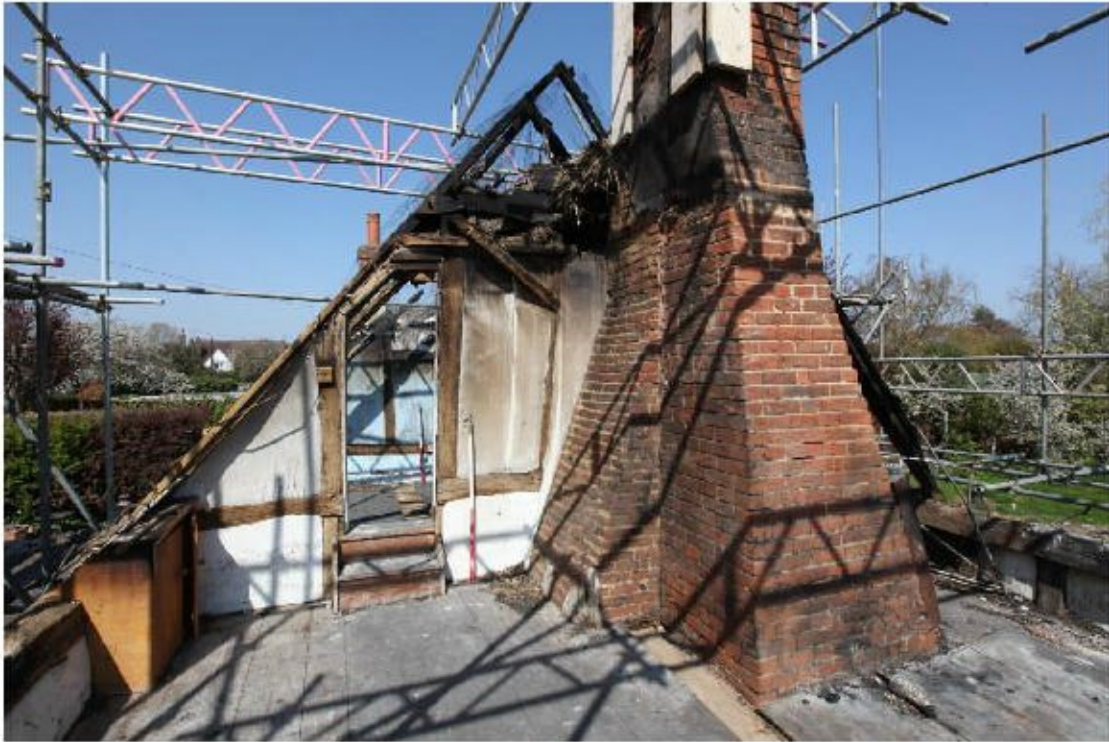
Illus. 31. The probable service chamber from its south-eastern gable showing the 19 th century brick chimney against its late-16 th or early-17 th century predecessor. Part of the probably original roof structure survives to the left of the chimney as shown in illustration 32.
