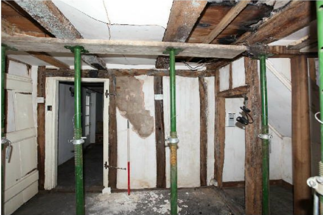
Illus. 13. The service bay from its rendered north-western gable showing the framed original door to the central hall on the left with an external door alongside. The wide spacing of the ceiling joists in front of the hall door indicates the position of a former stair but there is no firm evidence of an original stair trap.
