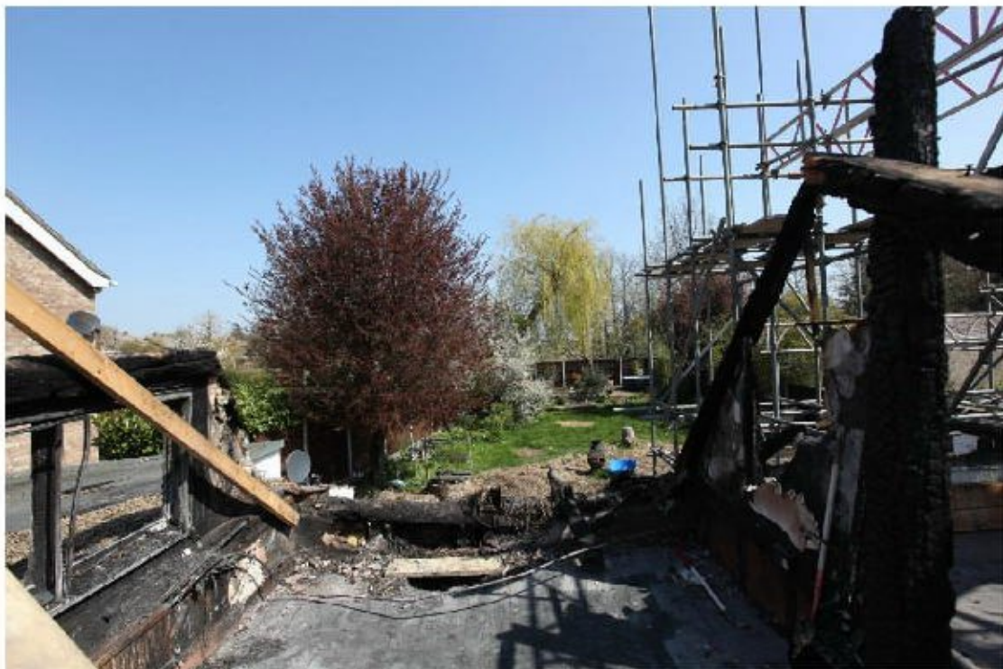
Illus. 26. The north-western chamber from the south-west showing the charred but intact rear roof-plate hidden by plasterboard and modern iron straps.
