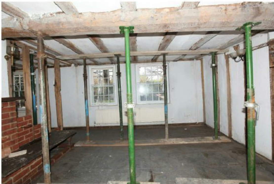
Illus. 6. The front (south-western) wall of the central hall showing its rendered brickwork and sash windows with the modern fireplace to the left. The hall extends to only 3.8 m in length (12.5 ft), but the original fabric of its external walls is either lost or hidden.
