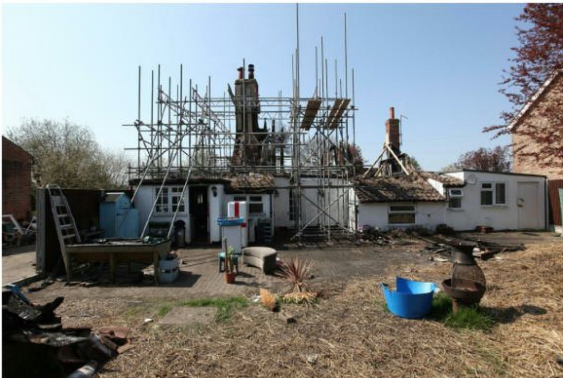
Illus. 4. The north-eastern elevation from the rear garden showing the two pantiled lean-to additions behind the modern kitchen in the parlour bay on the left and the original service bay to the right – much as shown on the 1875 Ordnance Survey. Most if not all of the garage to the extreme right is a 20 th century extension.
