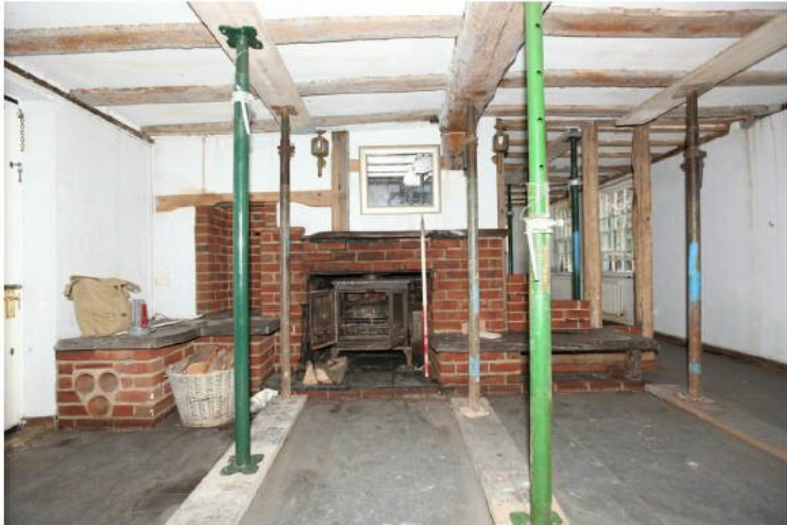
Illus. 7. The south-eastern wall of the central hall showing the 20 th century brick fireplace and wood-burning stove in the original chimney with a gap in the later studwork for a connecting door to the parlour on the extreme right. The recess on the left appears to represent part of the original fireplace.
