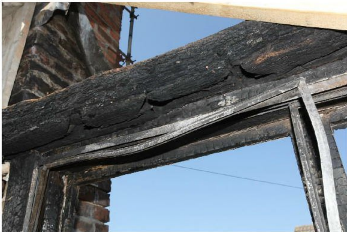
Illus. 24. A detail of the upper tie-beam of the north-western internal gable (illus. 23) showing empty mortices for three diamond window mullions with a groove for an internally sliding shutter.
