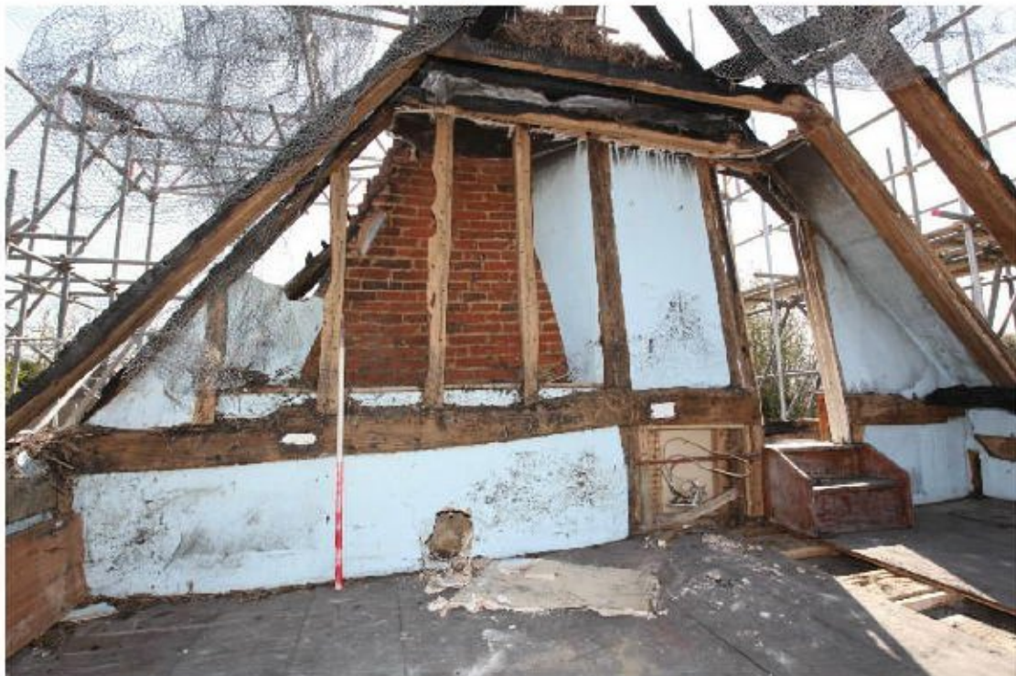
Illus. 30. The partition against the chimney at the south-eastern end of the hall chamber with an inserted door to the parlour chamber cutting the tie-beam on the right. The tie-beam contains pegged mortices for original studs with wider gaps for an original ground-floor door or doors to the right. The present studs above the tie are later insertions but it contains pegged mortices for original framing at least in the centre. See figure 14.
