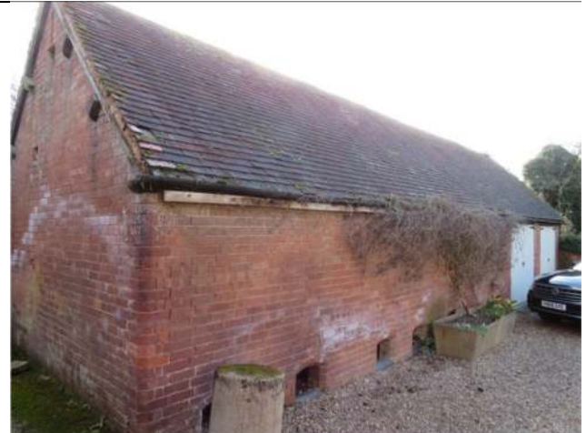
Photograph 2. The west and north elevations of the Barn
