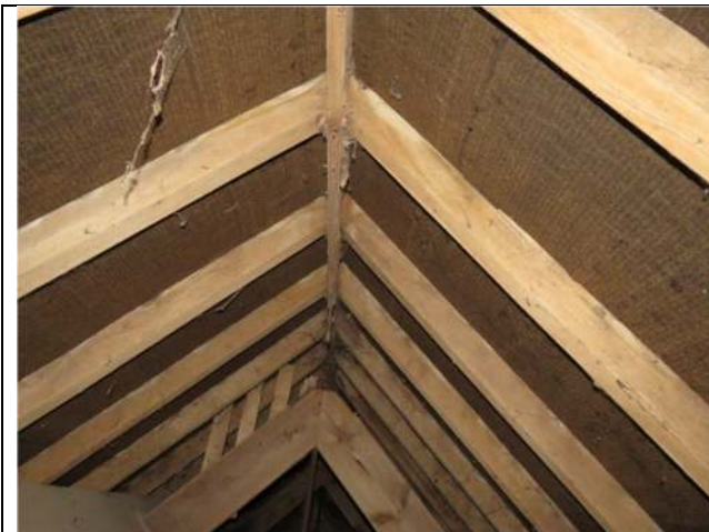
Photograph 9. Exposed timbers within the bat loft
