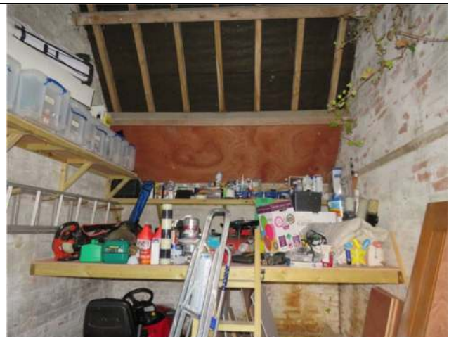
Photograph 10. The most southerly room within the Barn
