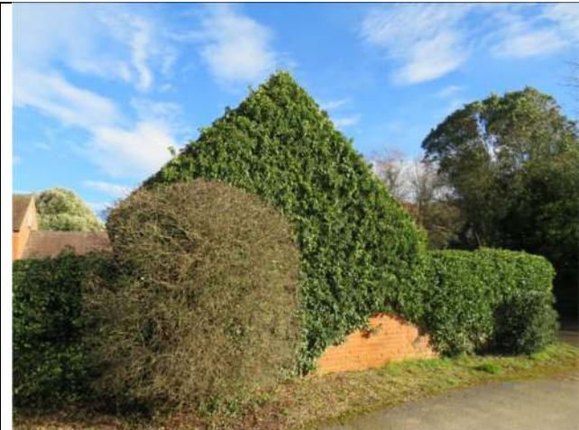
Photograph 3. The south elevation of the Barn
