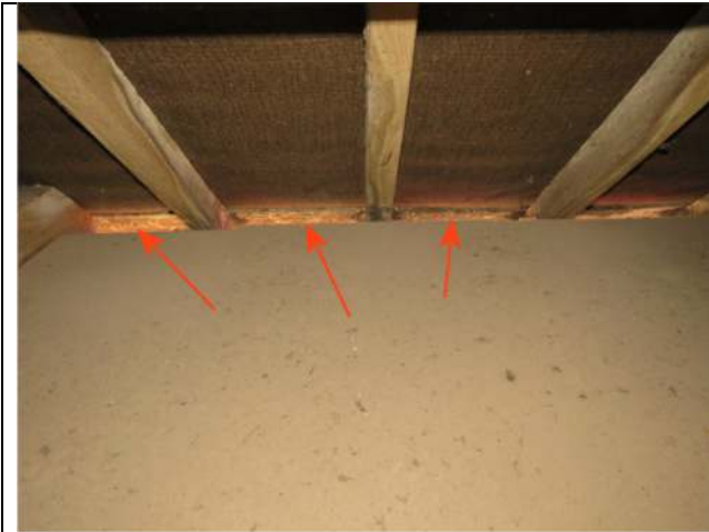
Photograph 7. Access into the Barn via the eaves openings between rafter tails
