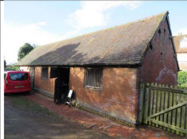
Photograph 1. The east and north elevations of the Barn
