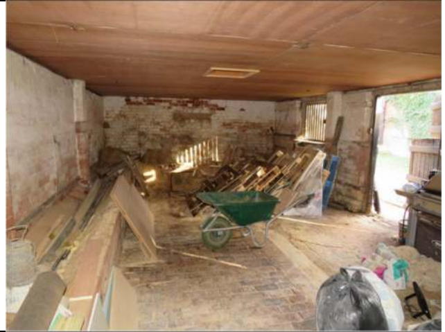
Photograph 14. The ground floor area within the Barn below the 'bat loft'
