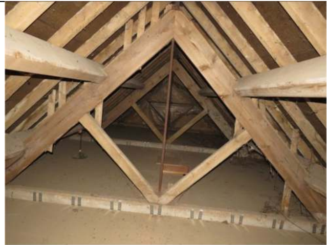
Photograph 8. The interior of the 'bat loft'
