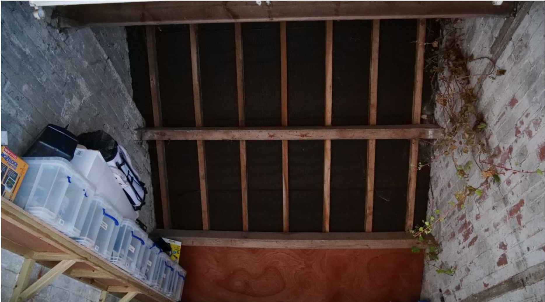
Figure 25: View of Cartshed Purlins and Rafters – with indication of modern re-roofing
