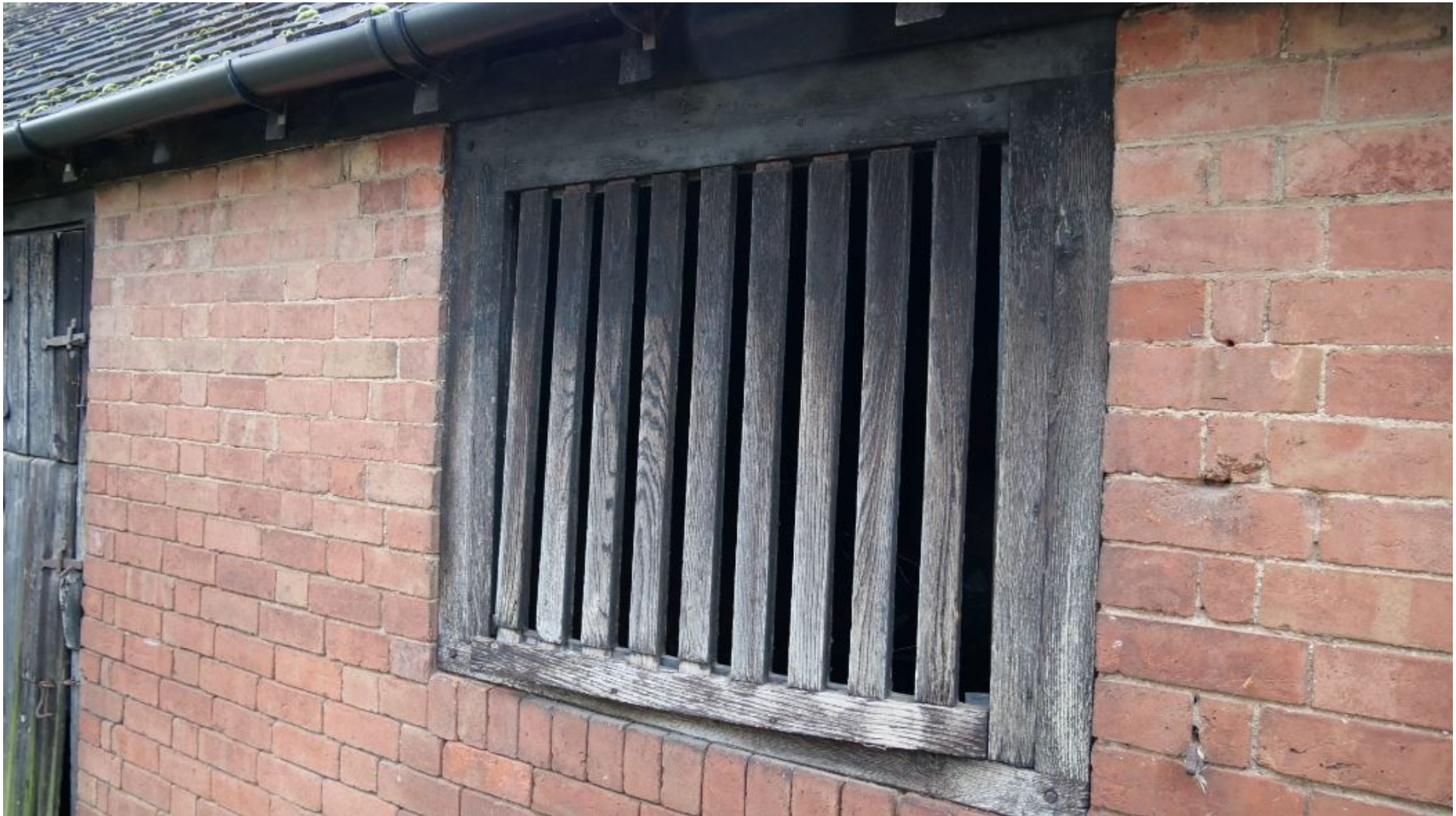
Figure 16: View of Cowshed Window Grille
