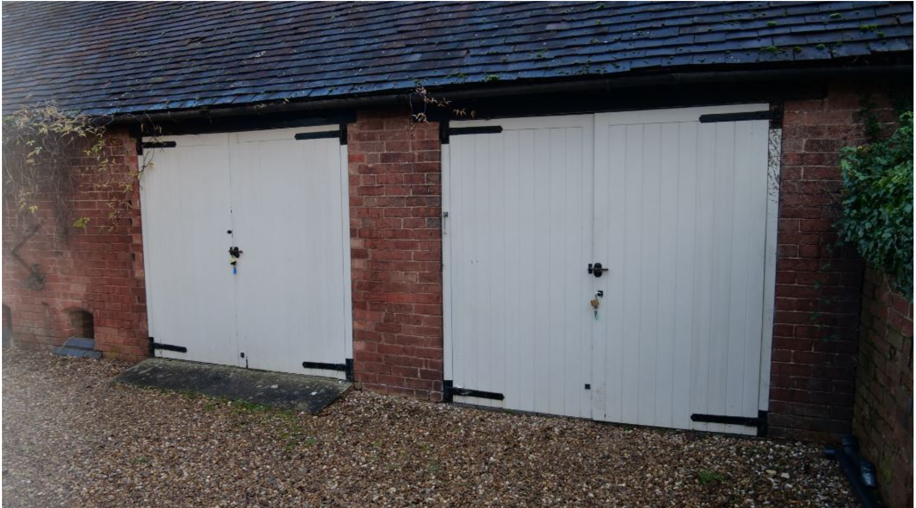
Figure 22: View of Two Door Openings on Eastern Elevation of the Barn
