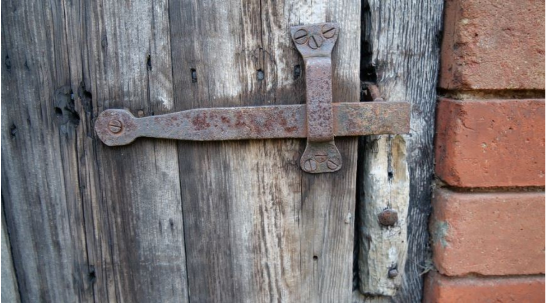
Figure 15: View of Original Handmade Simple Stable Door Latch – likely to be later provenance than other latch with cross motifs
