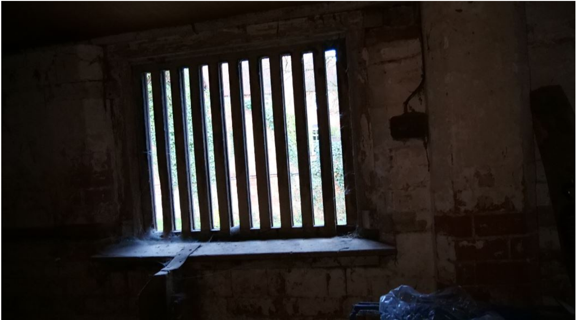
Figure 17: Internal View of Cowshed Window Grille
