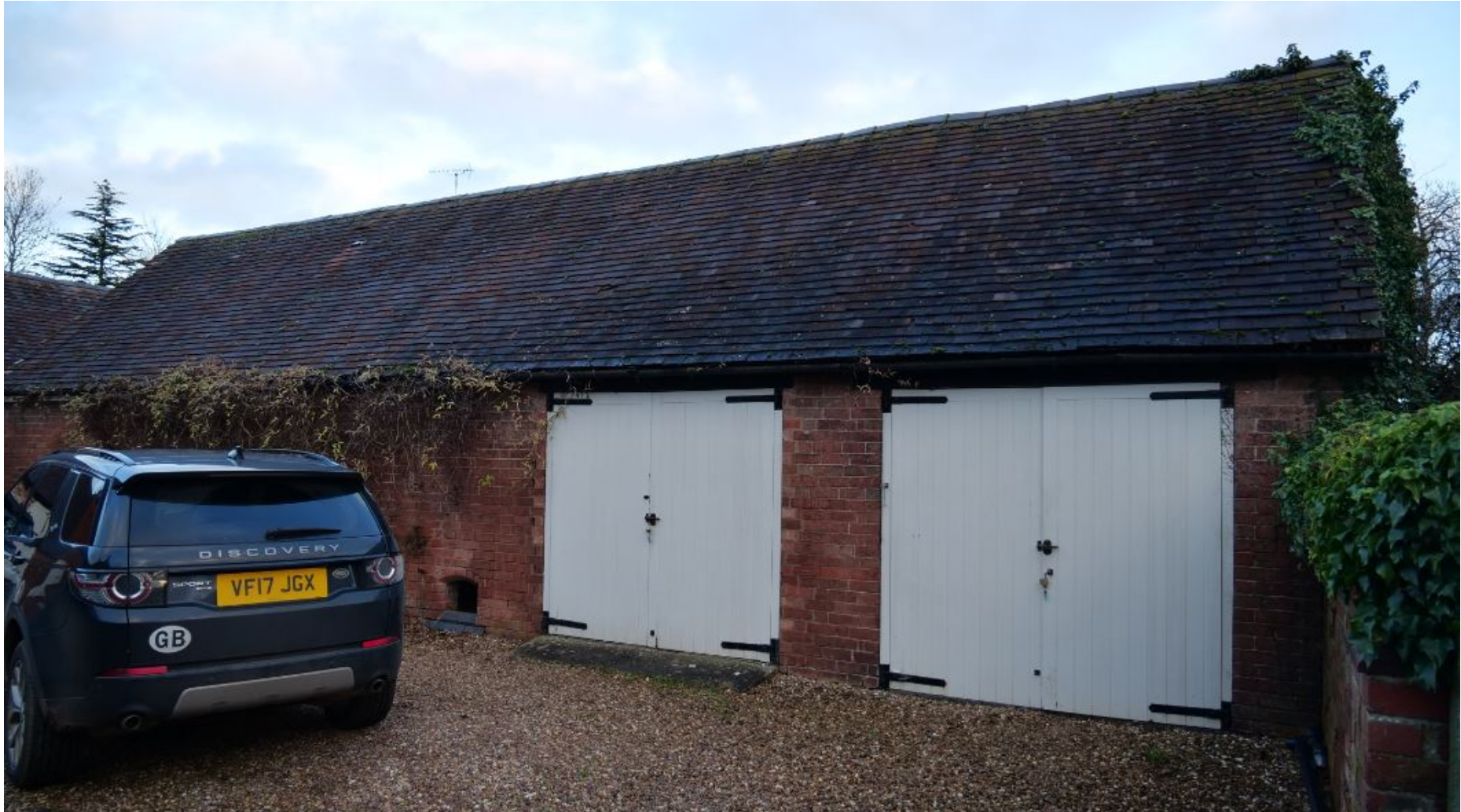
Figure 9: View of Barn Western Elevation – White Doorway on the right is in an original opening for a Cartshed and the door on the left is a new late C20 insertion with raised floor
