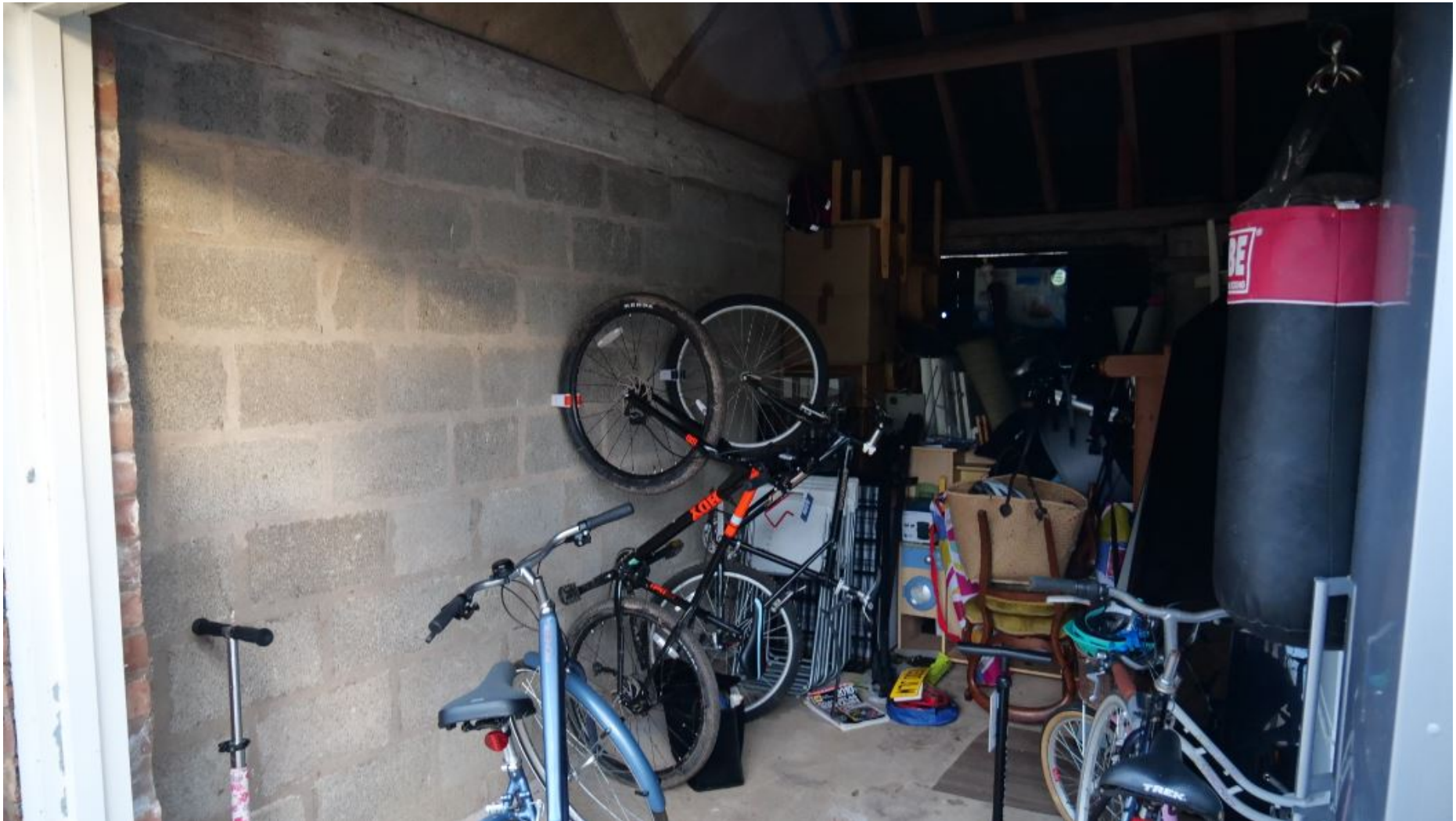
Figure 28: View of C20 Garage with new Blockwork wall
