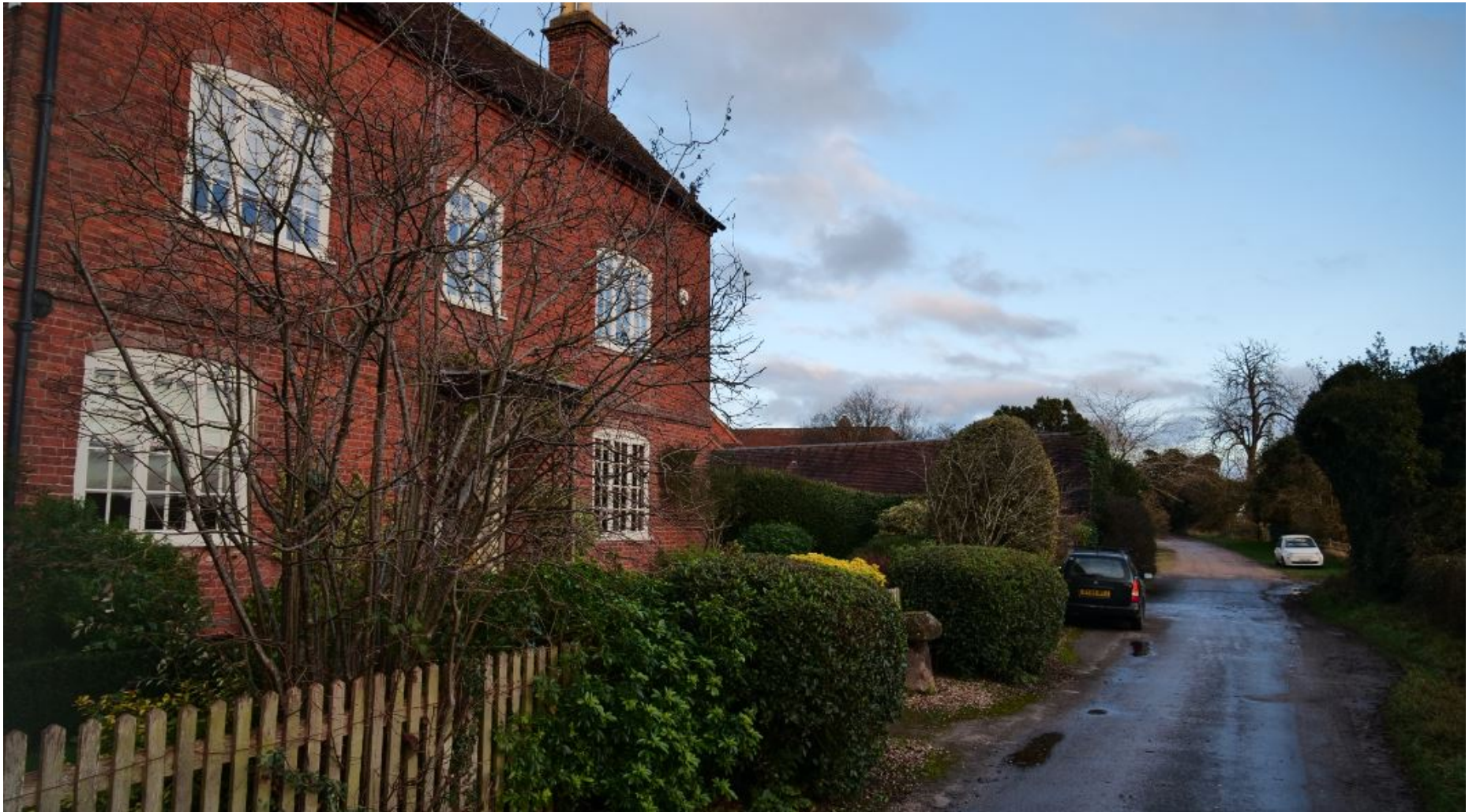
Figure 4: View of Grove Farmhouse with Curtilage Listed Barn and other Outbuildings behind
