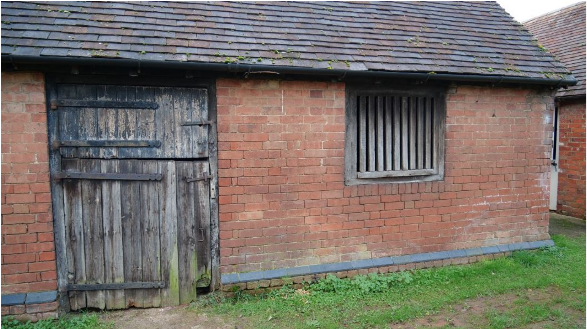
Figure 12: View of Eastern Elevation Stable Door and Window
