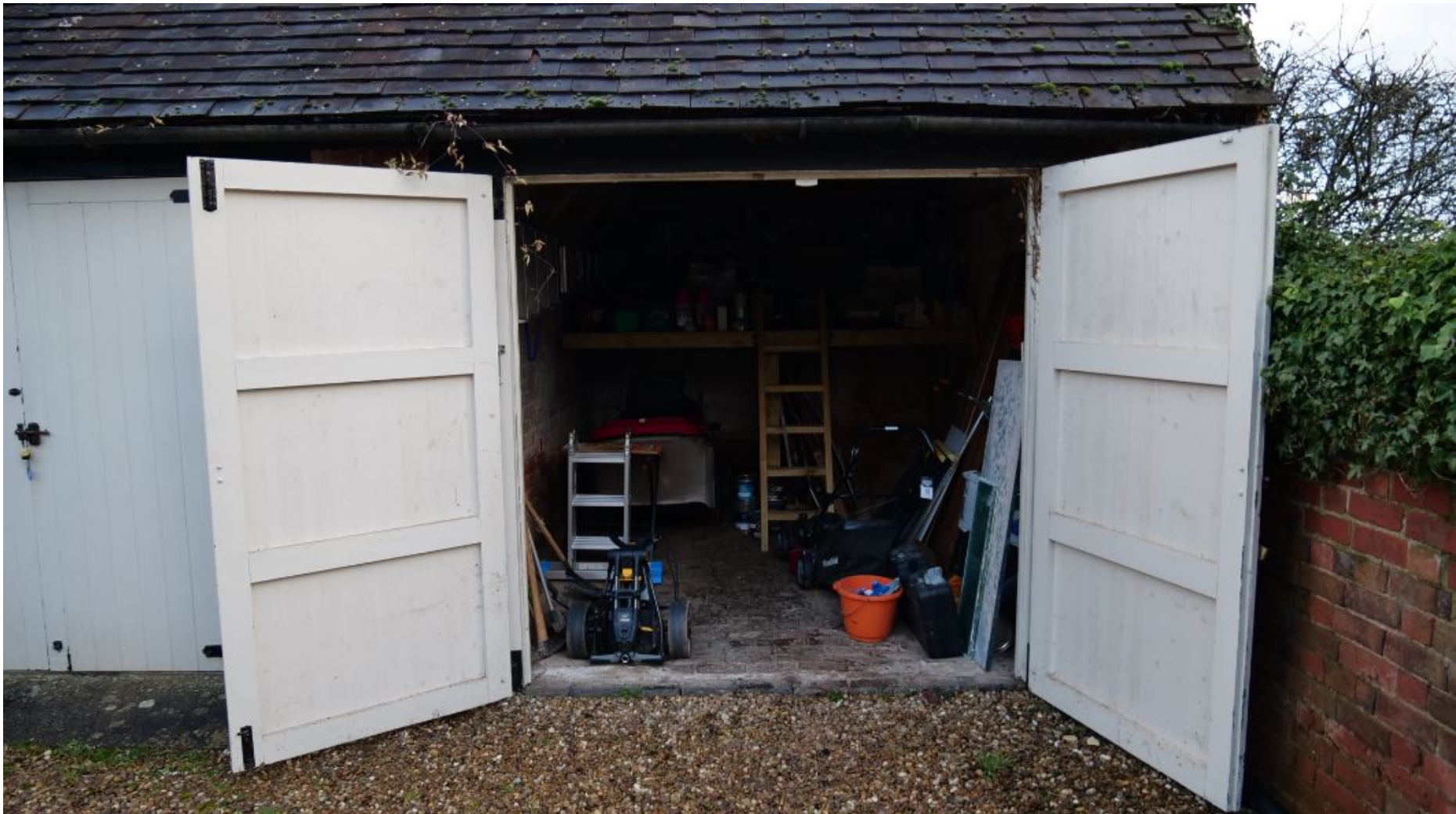
Figure 23: View of former Cartshed with modern Doors
