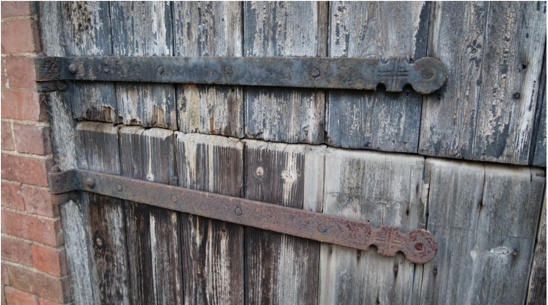
Figure 13: View of Original Stable Door Hinges with Cross Motif in Metalwork
