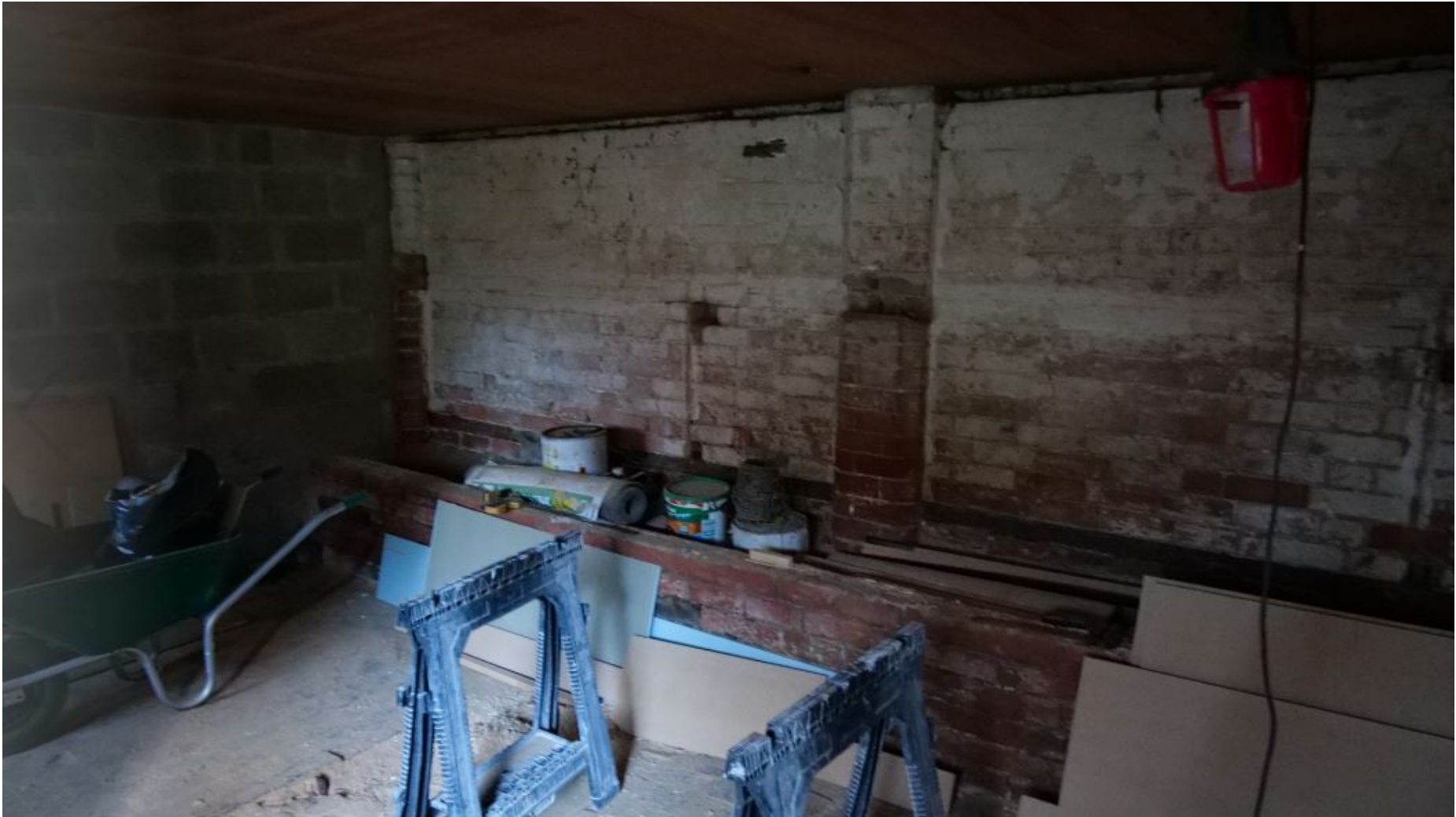
Figure 33: View of Cattle Feeding Trough – with Hen Nesting Holes Constructed Beneath
