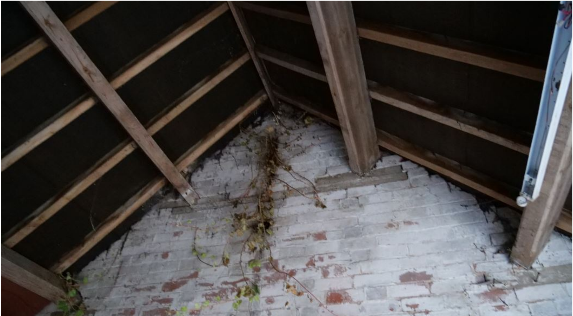
Figure 26: View of Cartshed Purlins and Rafters – and roadside gable brickwall
