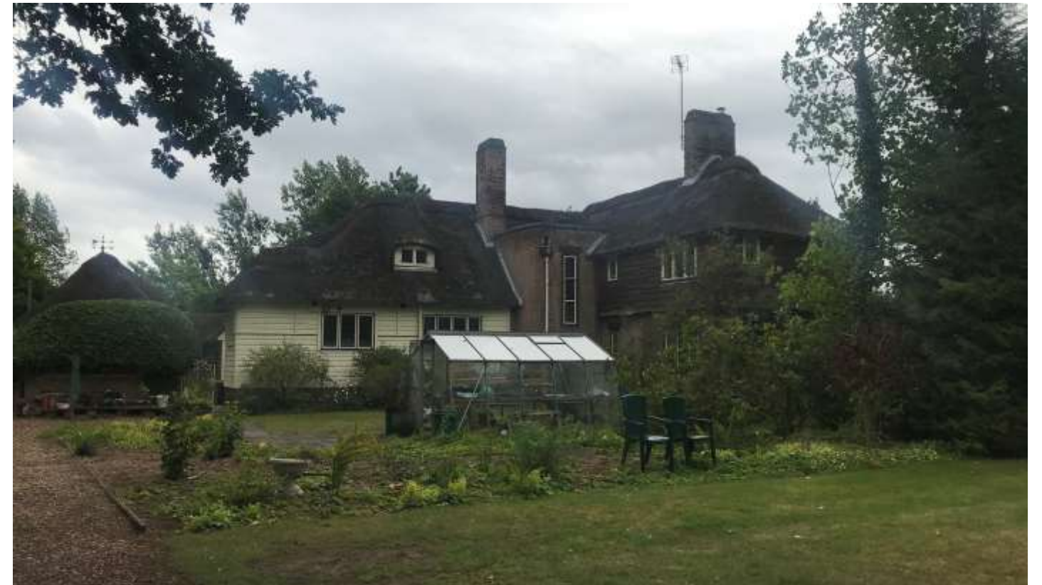
Photo 6: View of Arrow Cottage from north (service end of the garden, includes the greenhouse)
