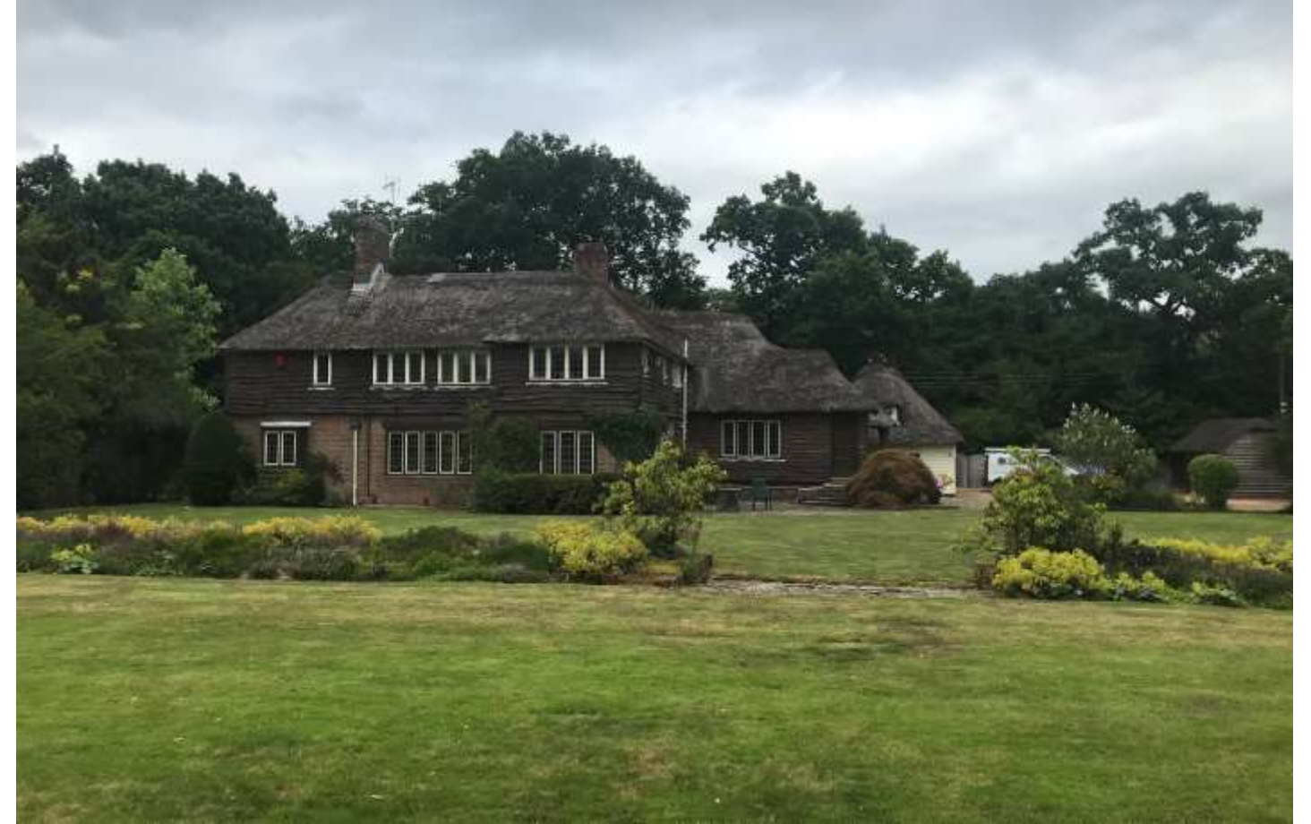
Photo 4: View of Arrow Cottage from south west (facing the formal garden)
