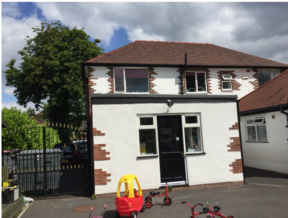
Figure 1 - existing rear elevation
