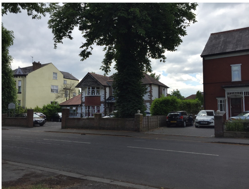
Figure 2 showing 35 Irlam Road (centre), a two storey building sited between two 3 storey dwellings.
