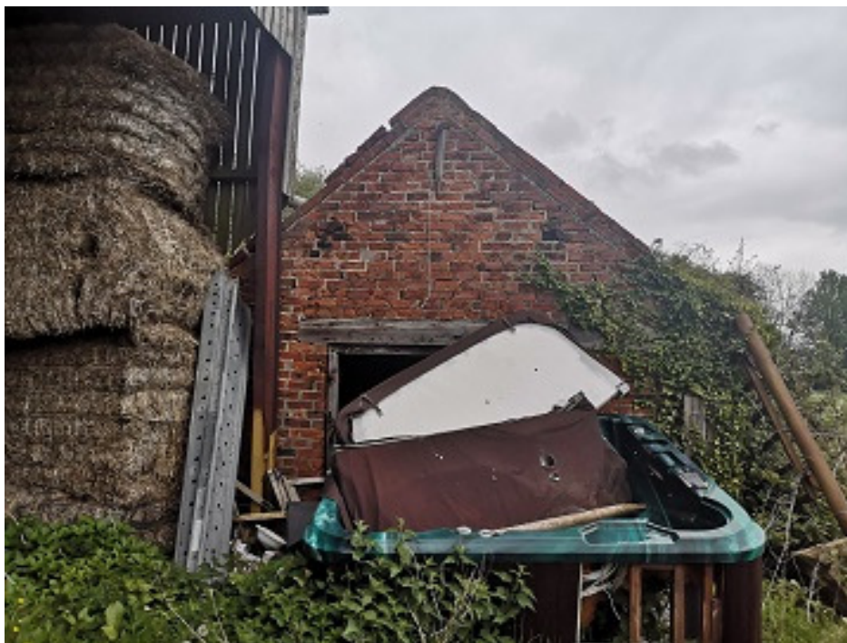
Plate 16. The west gable of Building 10.
