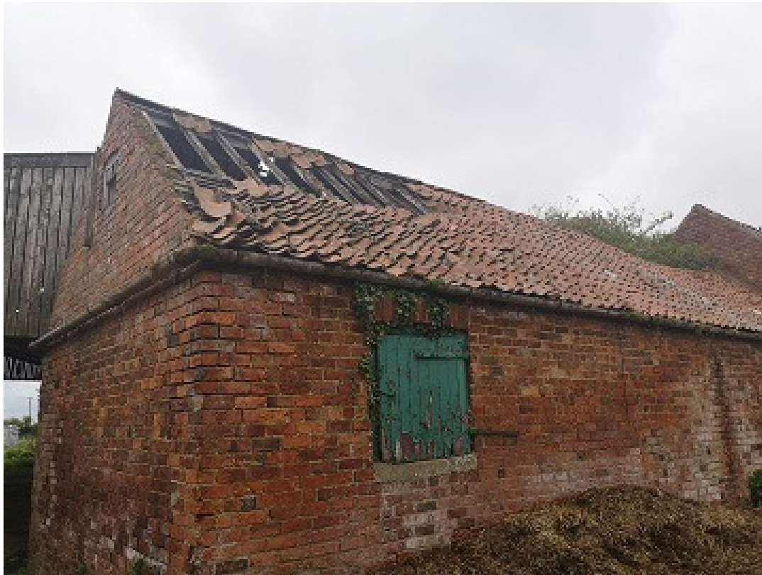
Plate 9. The north elevation of Building 6.
