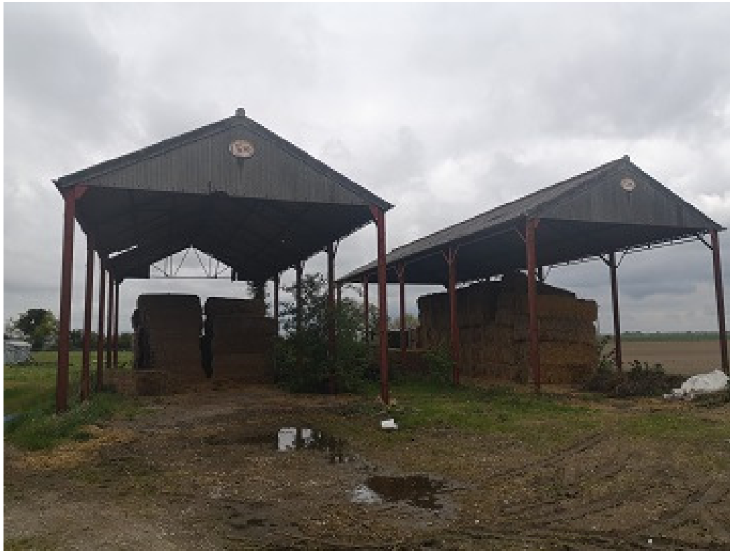
Plate 3. Looking toward the north gables of Buildings 2 & 3.
