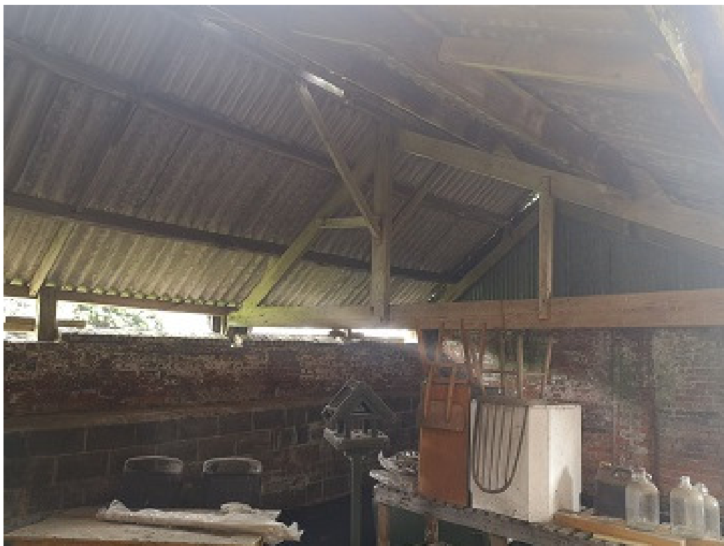
Plate 15. Looking east into Building 9 from the interior of Building 8.
