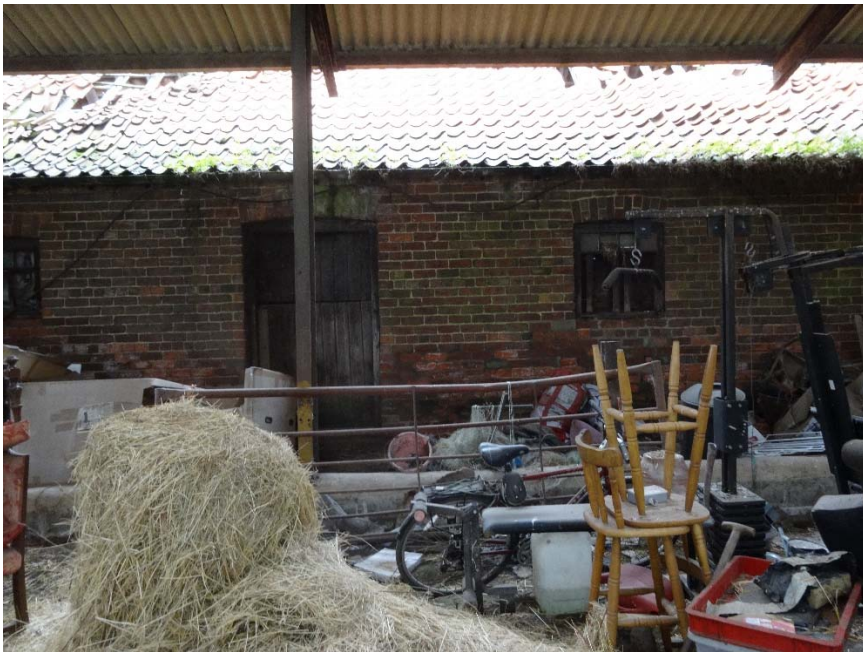
Note the window and door head brick arches all appear to be in good condition with no signs of fracture cracks.
