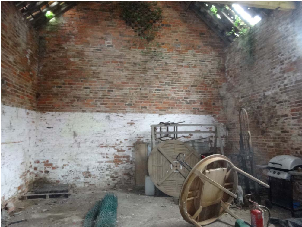
Internally the wall is well mortared and pointed and shows no signs of structural damage.
