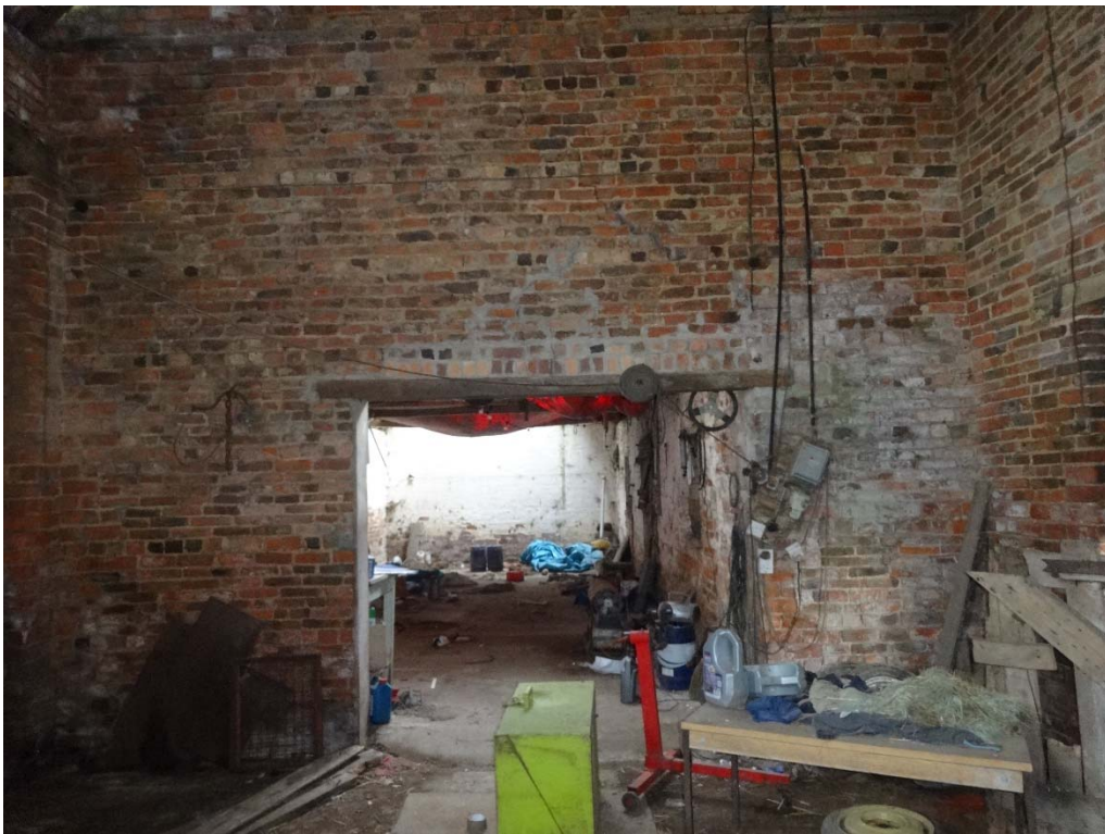
Internally the wall is well mortared and pointed and shows no signs of structural damage.
