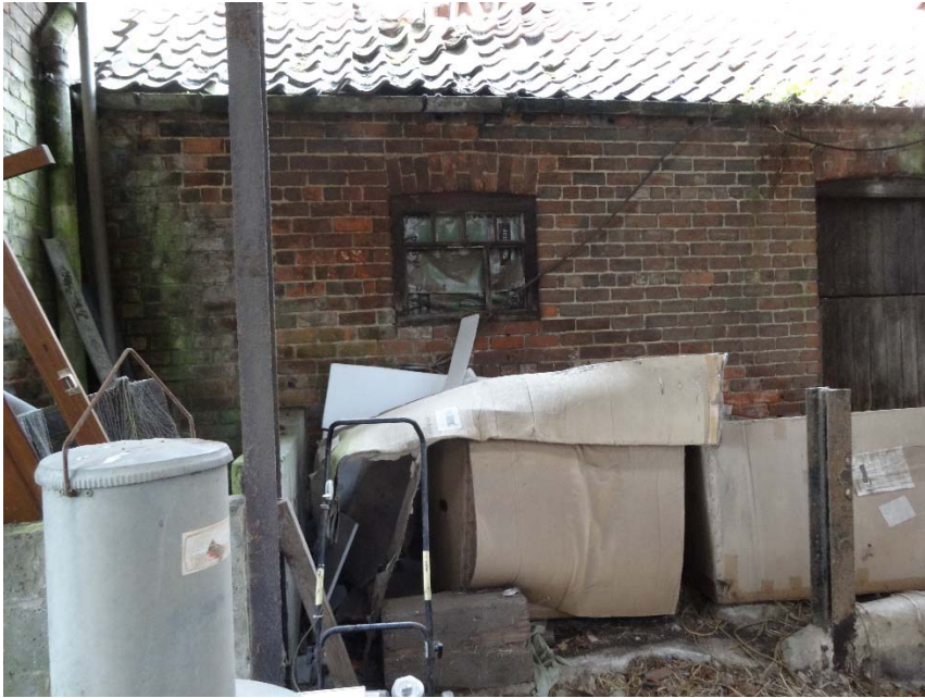
Note the window and door head brick arches all appear to be in good condition with no signs of fracture cracks.
