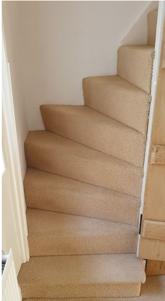
Photograph 3: Winder Staircase at no.17 Hollyhock Cottage
