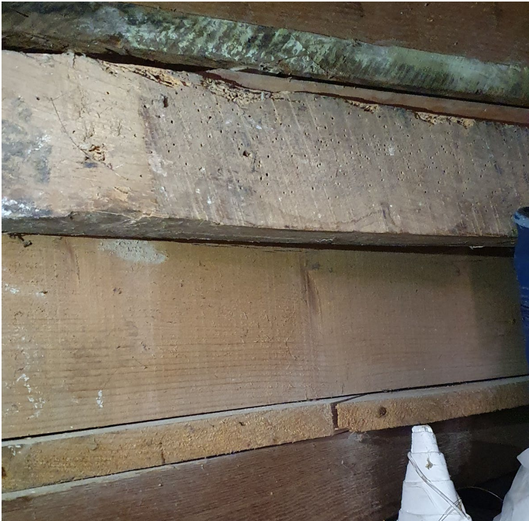
Photograph 6: Bearers Supporting the Winder Steps
