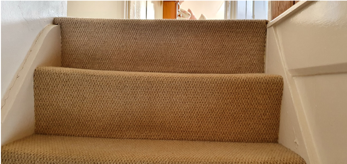
Photograph 4: Stair Strings Visible above the Stairs (to match skirting height)
