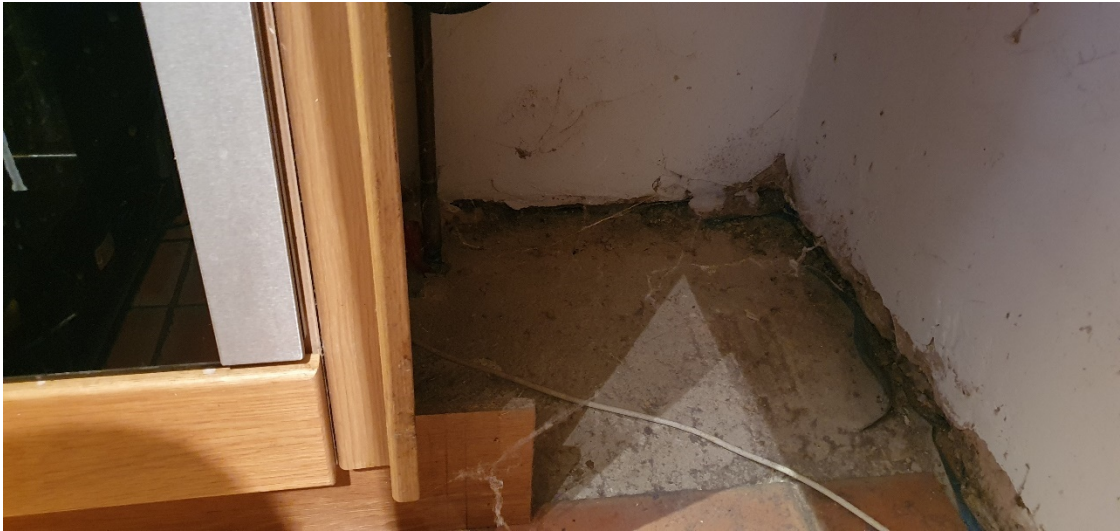
Photograph 2: Concrete Subfloor Exposed under Kitchen Units
