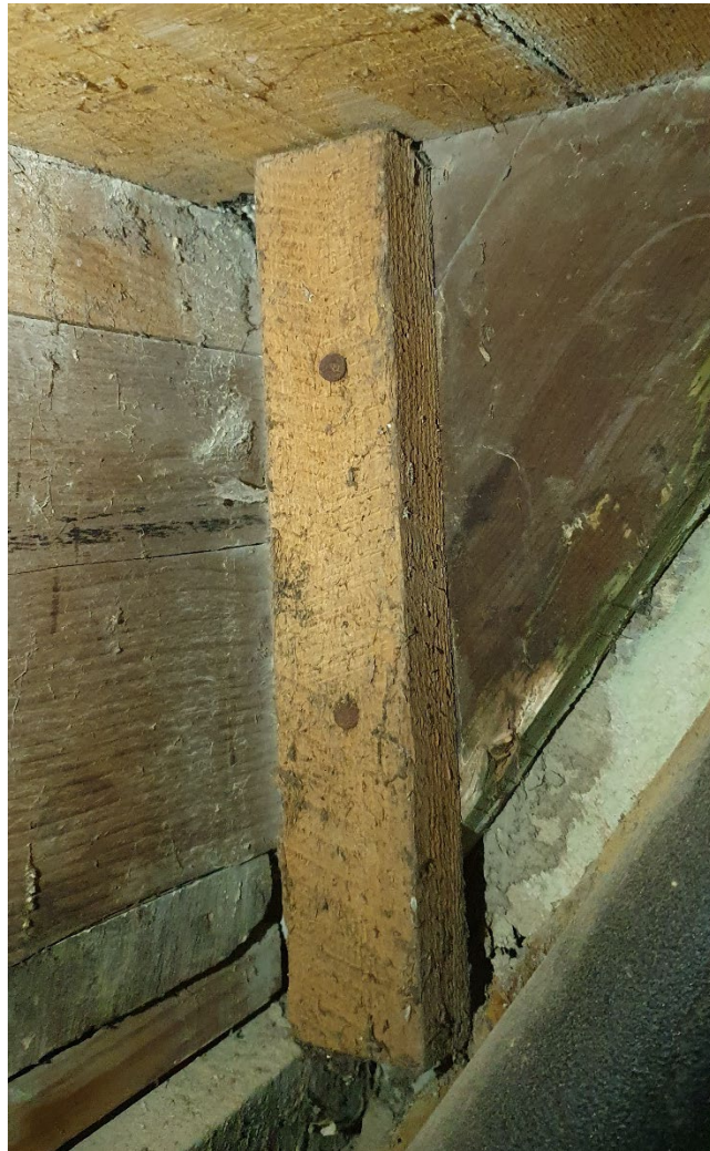
Photograph 11: Example of Unsympathetic Addition to the Staircase Construction
