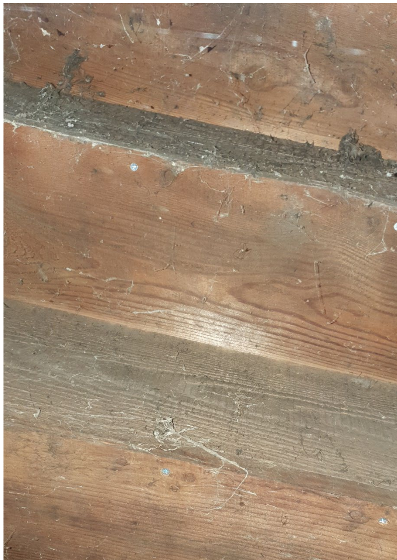
Photograph 9: Original Pine Staircase (note modern fastenings reinforcing the structure)
