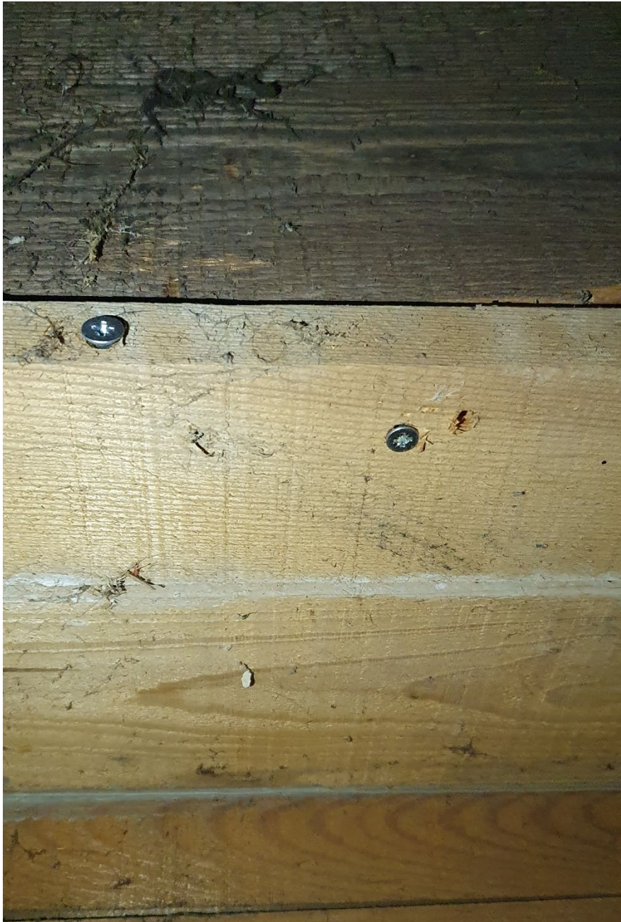
Photograph 12: Replacement Rough String
