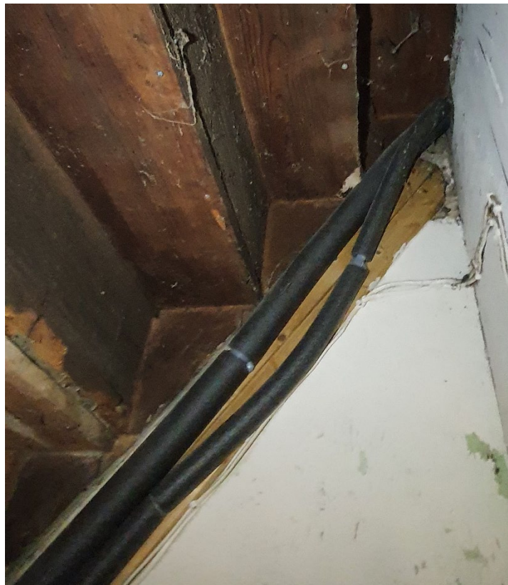
Photograph 5: Stair String Below Stairs
