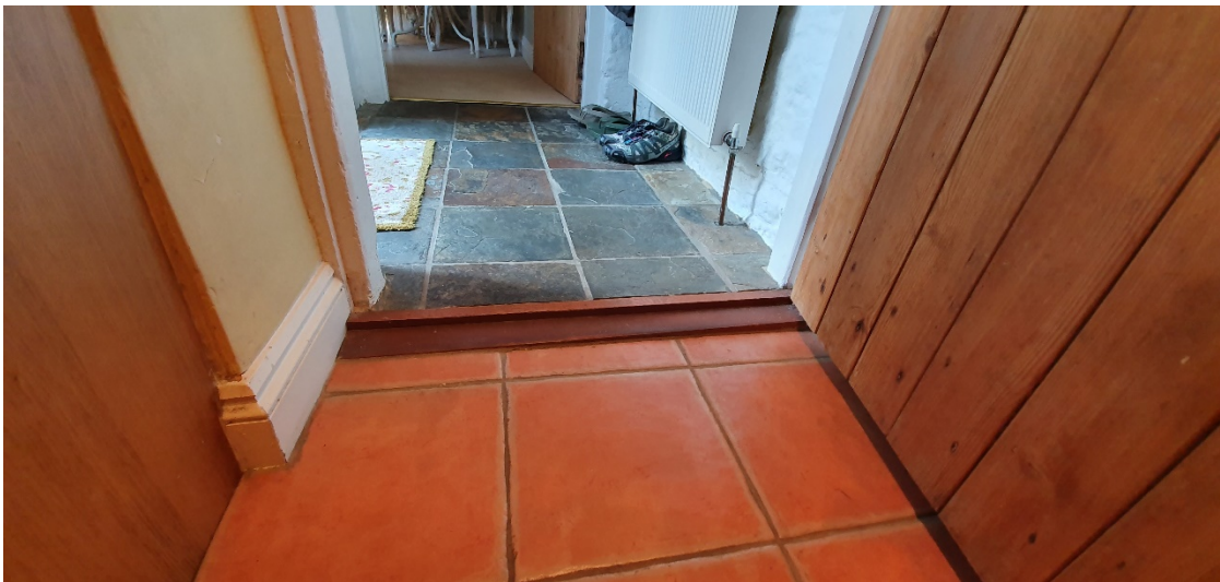
Photograph 1: Kitchen Floor Materials
