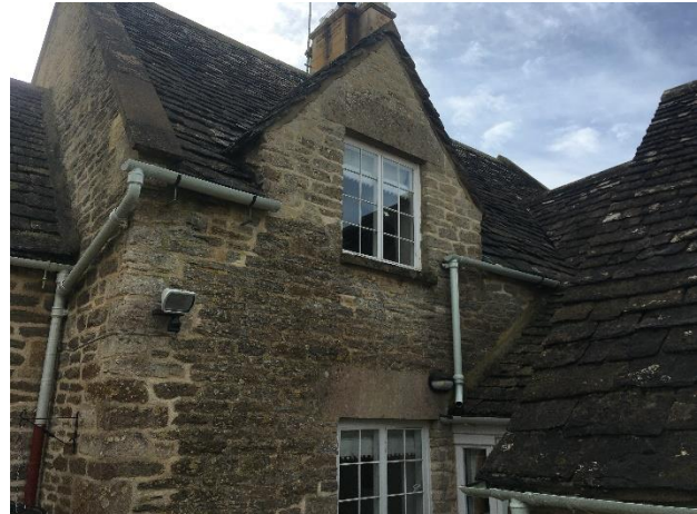
Figure 6 - North elevation of the house
