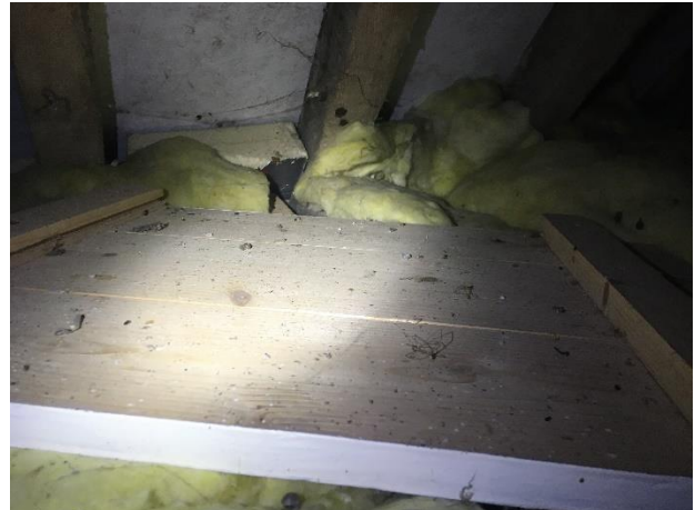
Figure 4 - Internal loft space
