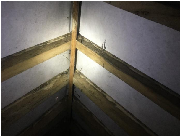
Figure 3 - Internal loft space
