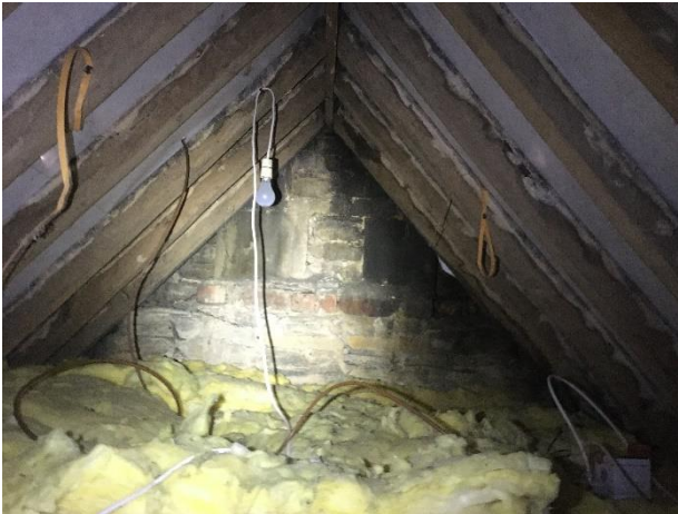
Figure 5 - Internal loft space
