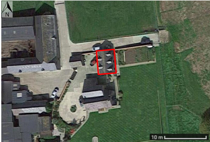
Close-up aerial photograph showing the site and building surveyed
