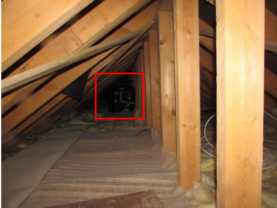
Plate 7 –Inside the loft of the building and location of water tank
