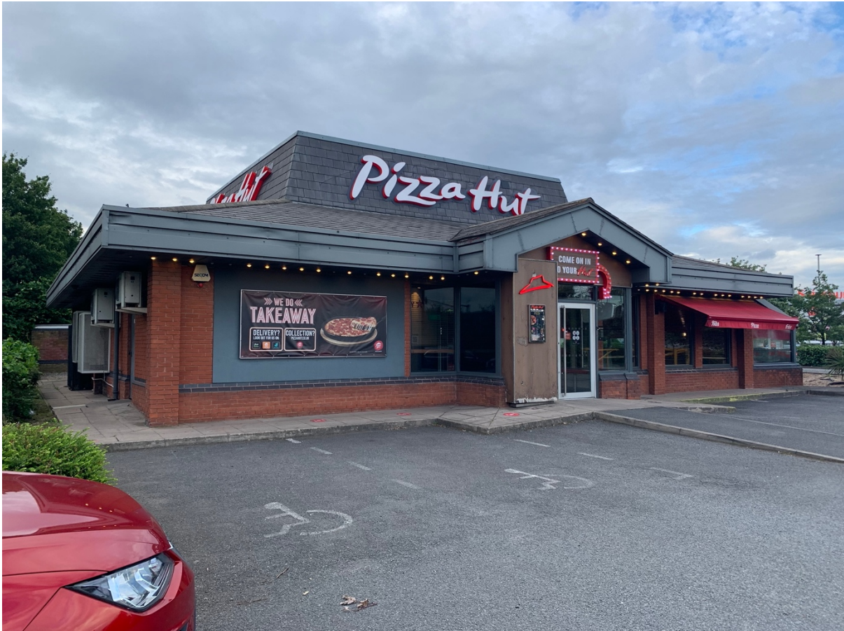
South Elevation – Main Entrance
