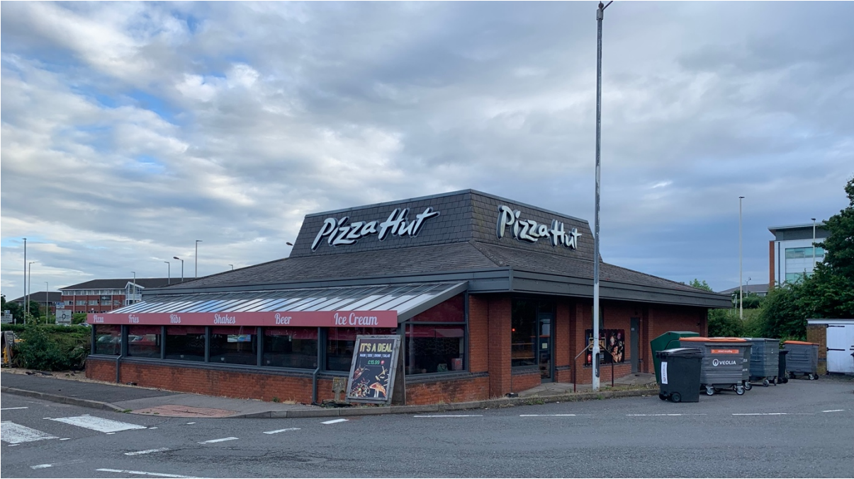
North and East Elevations – showing current service / bin store area
