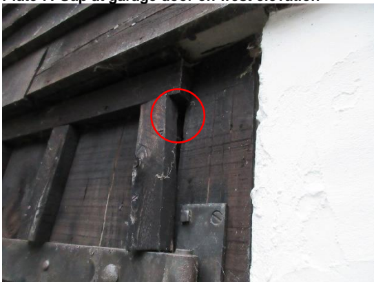
Plate 7: Gap at garage door on west elevation
