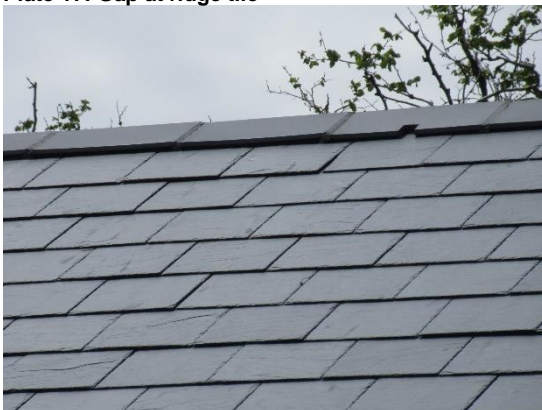
Plate 17: Gap at ridge tile
