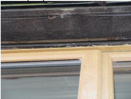
Plate 7: Gap at garage door on west elevation
