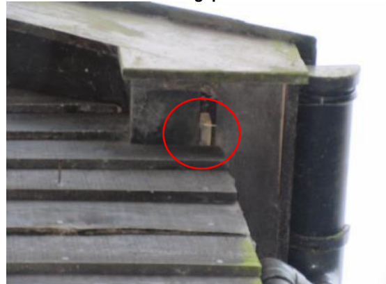
Plate 6: Gap at top of timber cladding
