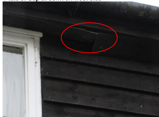
Plate 8: Gap at soffit on west side
