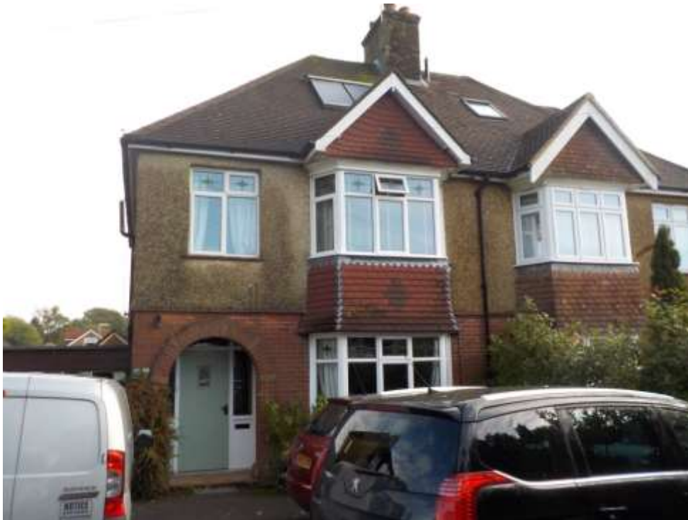
Photograph 01 – Existing South West elevation
