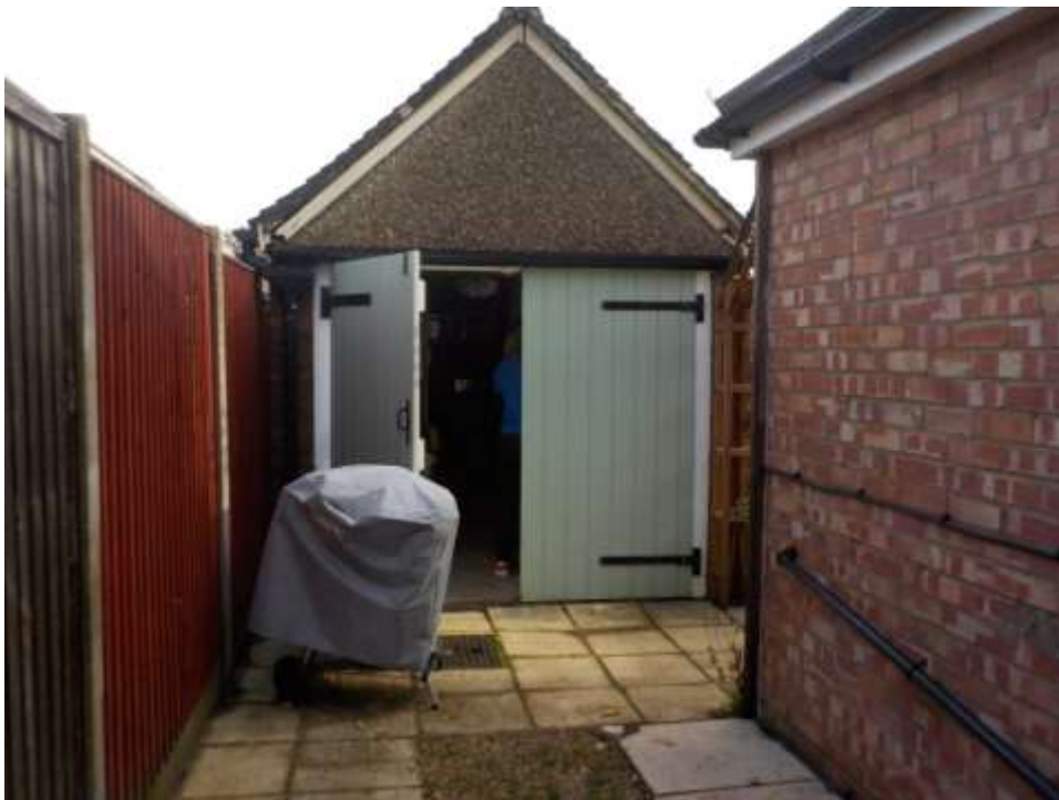
Photograph 03 - Showing the South West elevation of the garage
