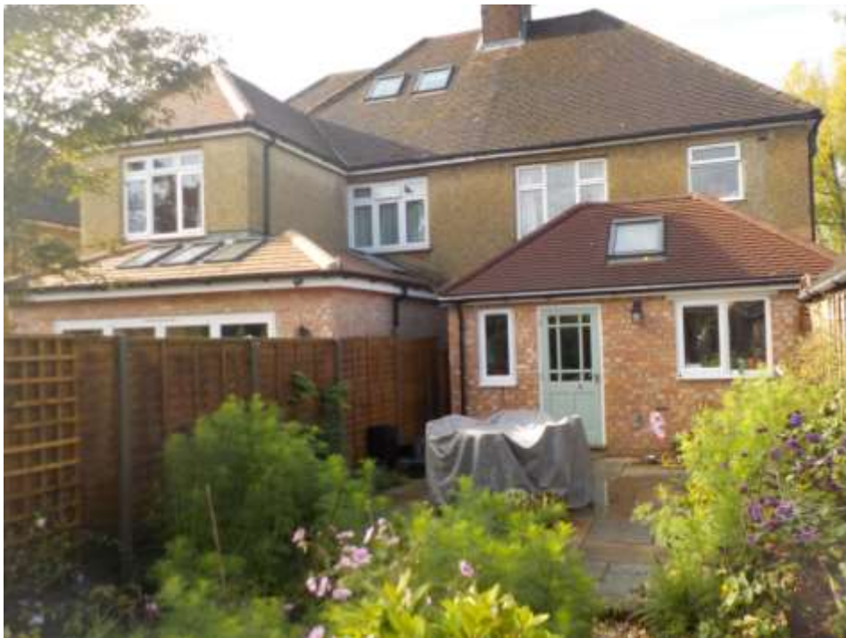
Photograph 02 – Existing North East elevation
